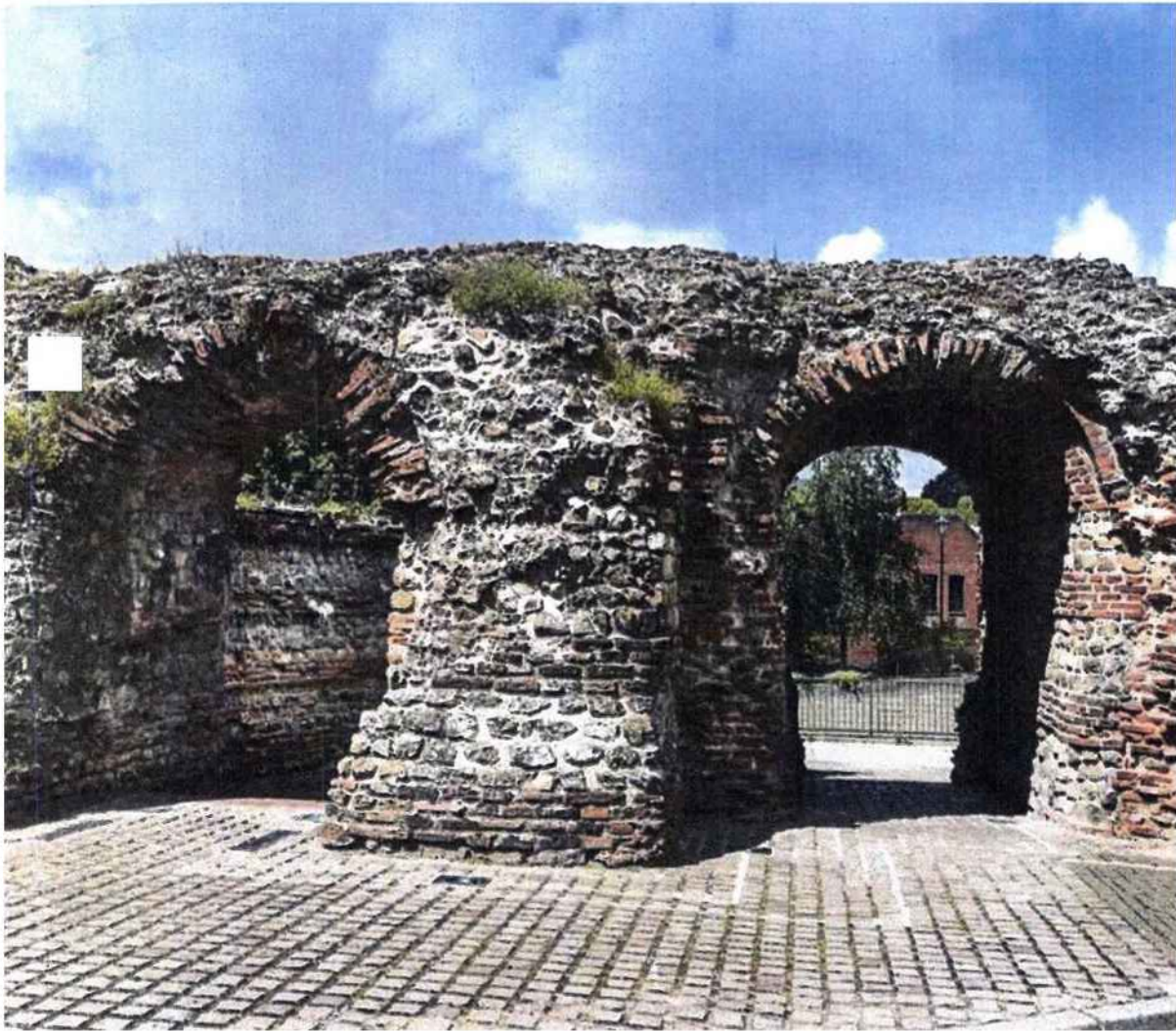
Fig.1 The surviving portion of the Balcerne Gate, Colchester, from inside the town. The walls are of flint and rubble stone, held together by bonding courses of brick and tile.
