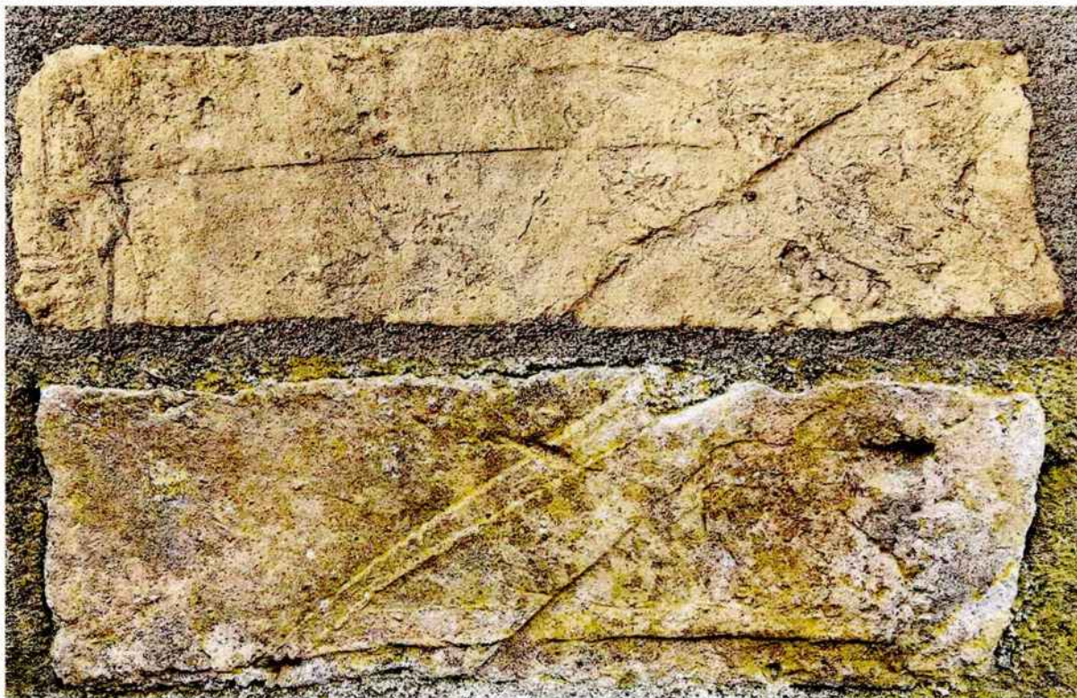
Fig.5 Two examples from Cambridge of bricks with more than one set of pressure marks.
