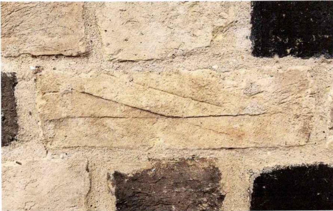
Fig.1 Restacked brick pressure mark on the stretcher of a brick found in the Garden Wall at Burleigh House, St Ives, Cambridgeshire. (Author)
