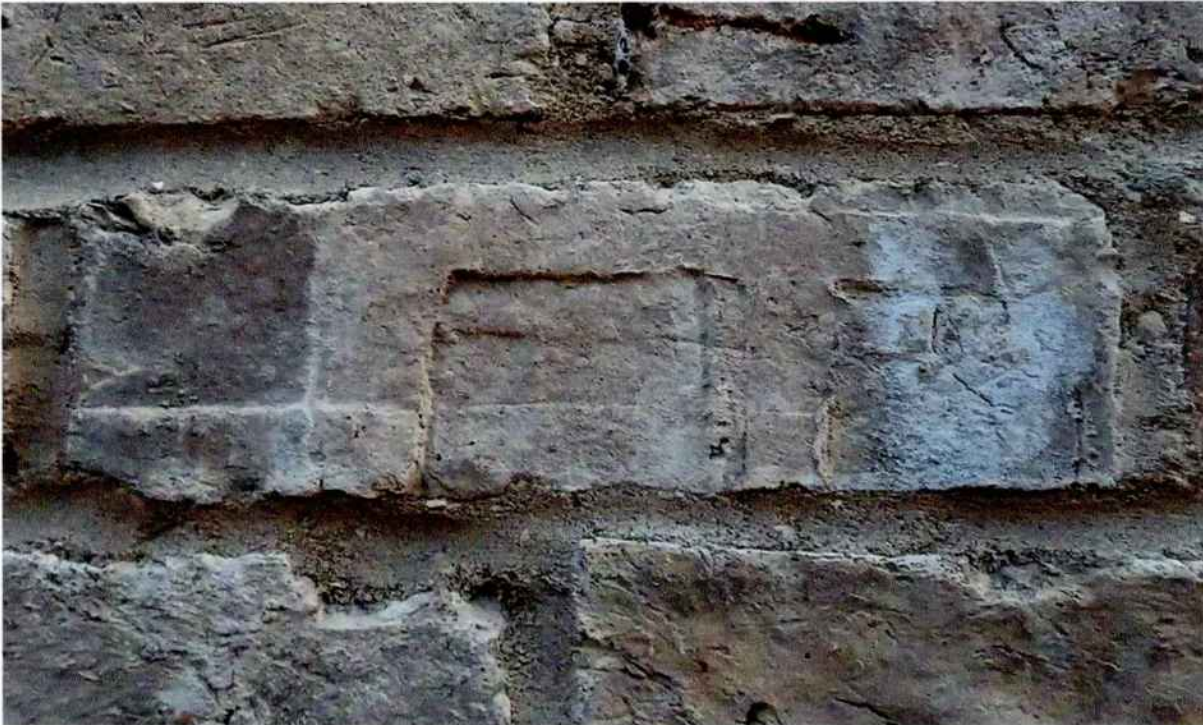
Fig.3 Wall at Kettle's yard showing horizontal, diagonal and vertical pressure marks. (Author)
