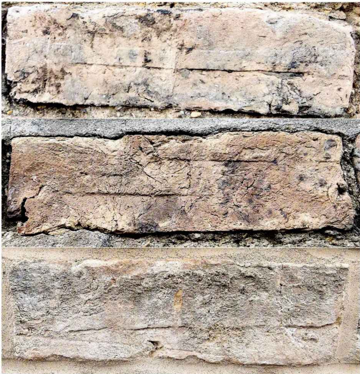
Fig.4 Examples of two pressure marks on bricks from Cambridge.
