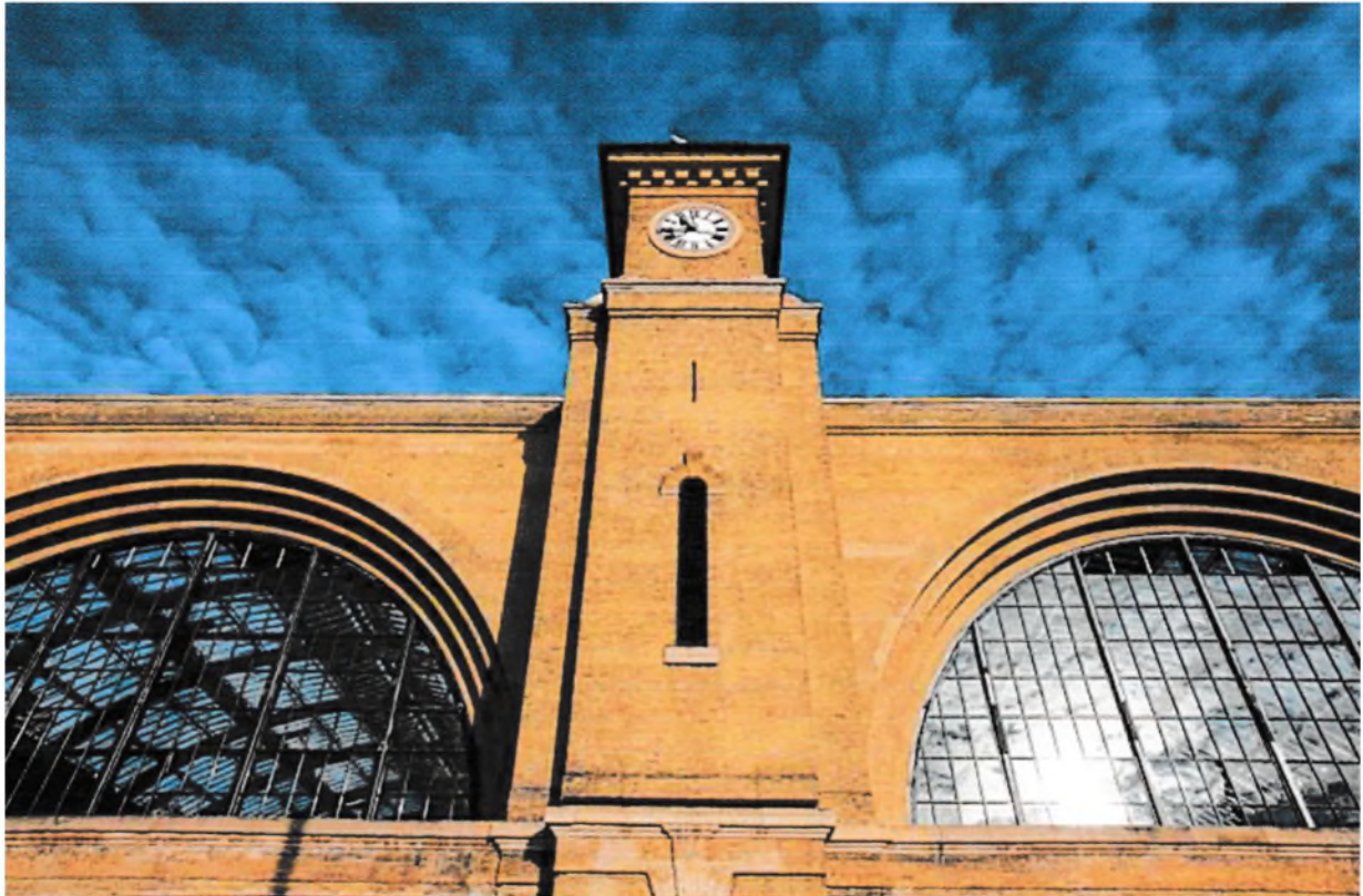
Fig.4 Kings Cross Station, the London terminus of the Great Northern Railway (later and at present the London and North Eastern Railway)
