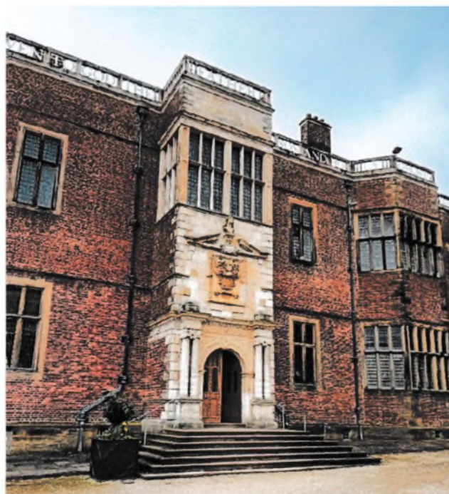
Fig.3 The Main Entrance, on the north Side of the South wing. The limestone cladding was added in the eighteenth century.
