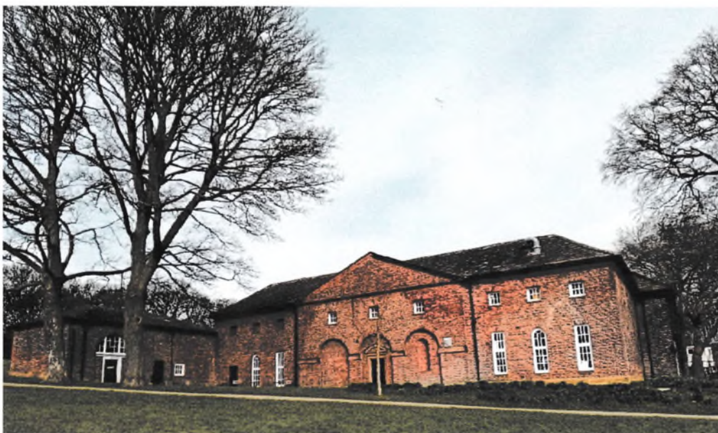
Fig.7 The West Front of the Stables, showing the later dairy to the left.
