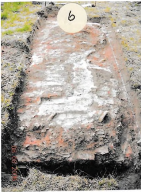
Fig.6.6 (left) Machine base with eight holding down bolts. Fig.6.7 (right) End section of the machine base.
