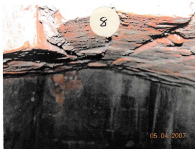
Fig.7.8 Internal view of the underground storage tank showing inlet hole.
