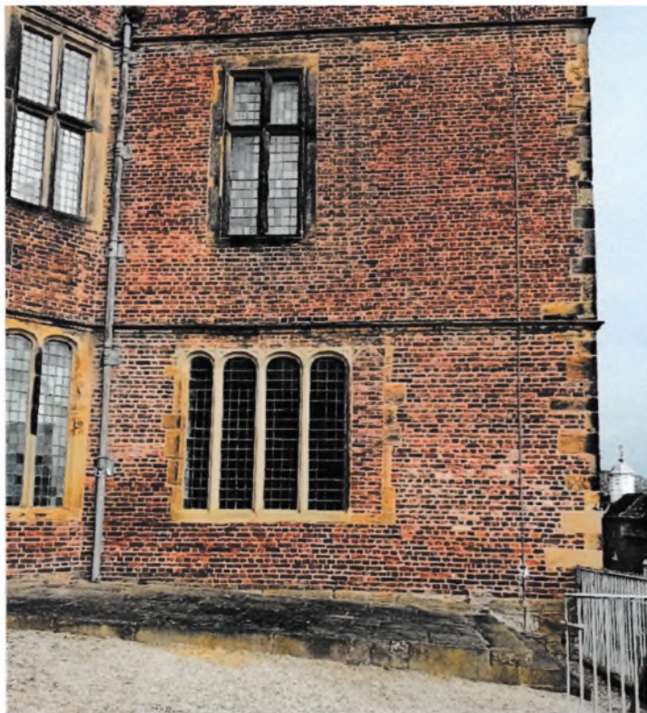
Fig. 4 Showing the alteration to the window of Sir Arthur Ingram's chapel, when it was later converted to a kitchen.
