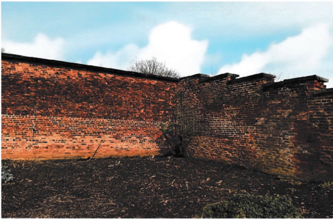
Fig.11 The angle between the South-facing and West-facing firewalls.
