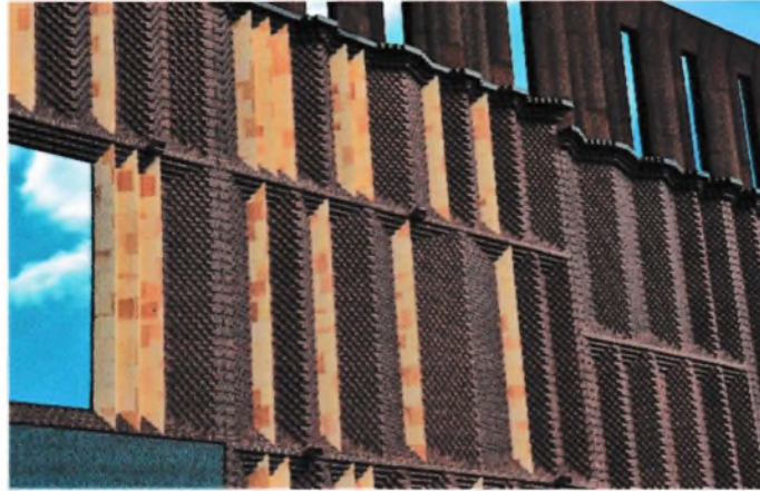
Fig.24 Award winning development, Victoria Gate, Leeds City Centre. A combination of Ketley brick slips and specials used to create an impressive façade.
