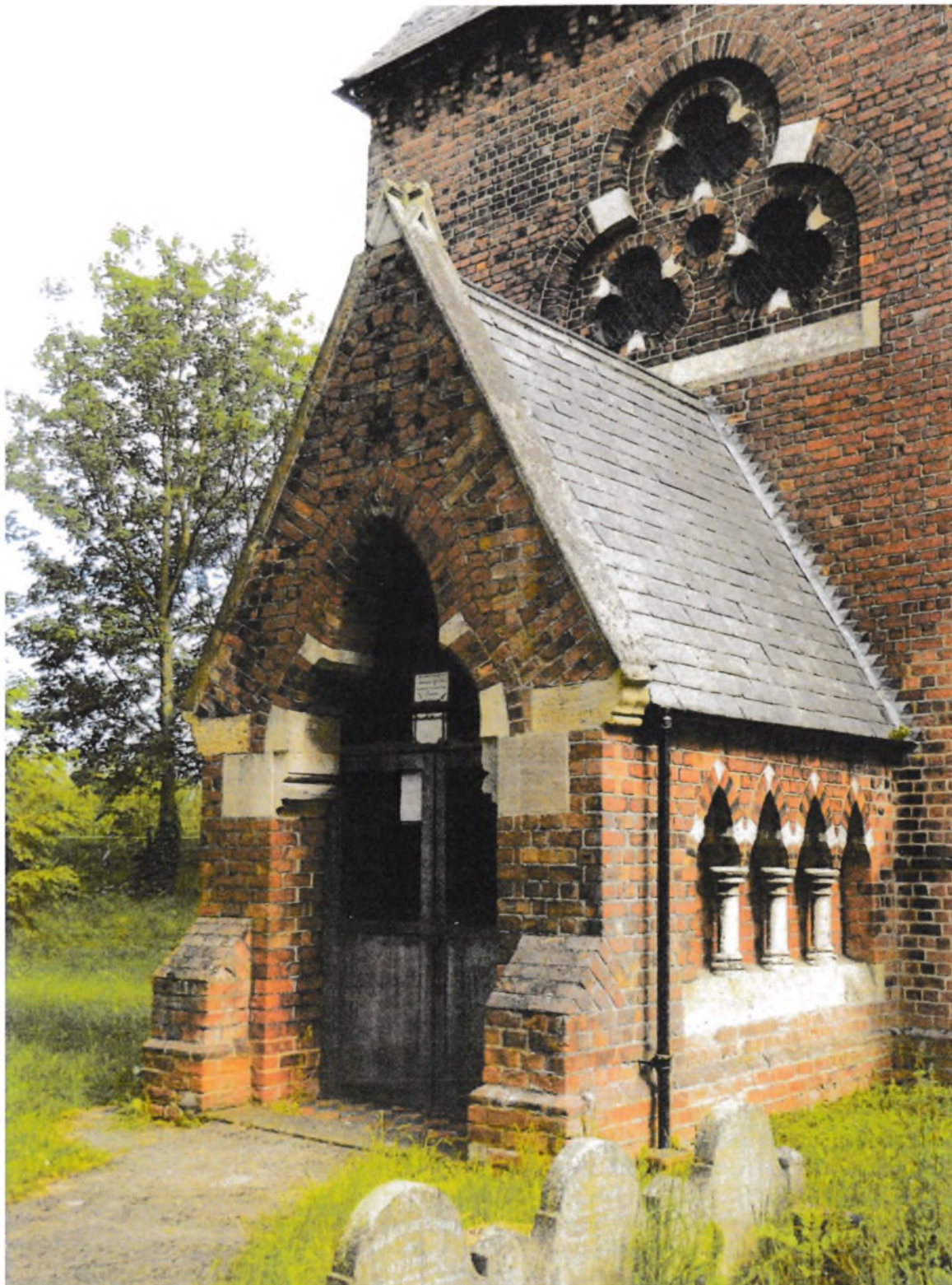
Fig.3 Burringham church: porch and tower. Note the use of the trefoil both in the upper part of the entry and in the window of the tower.
