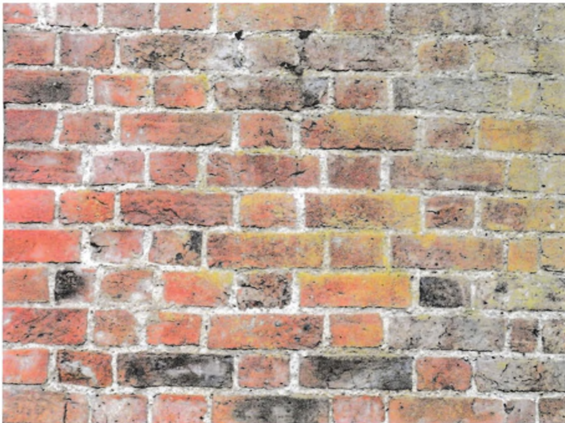
Fig.9 The blocking of the doorway of the eighteenth-century addition to the north side of the church was executed using machine-made bricks at a date after 1849. The brick are laid in English Bond. Photograph: Mike Chapman
