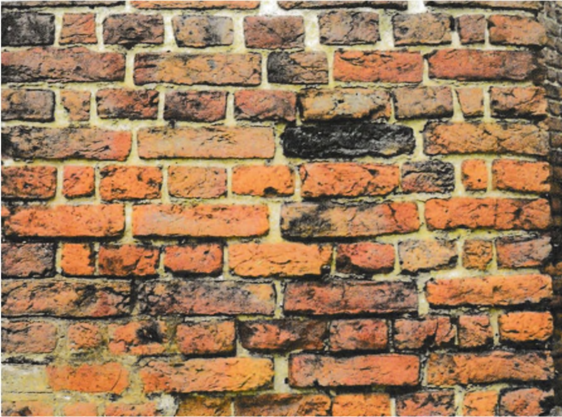
Fig.6 The main body of the church is red bricks laid in English Bond.
