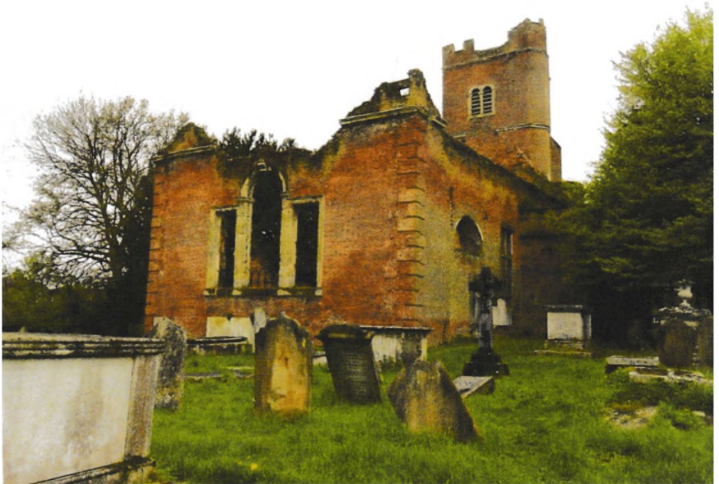
Fig.5 The surviving east wall of the 1632 brick church at Great Stanmore showing the Venetian window at the east end of the chancel space. Photograph: Mike Chapman
