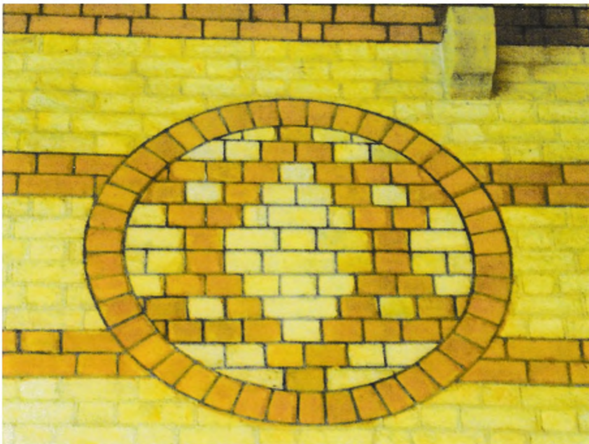
Fig.9 Burringham church: Seal of Solomon motif on the internal brickwork of the tower. (Both the shape and the colour are distorted in this photograph.)
