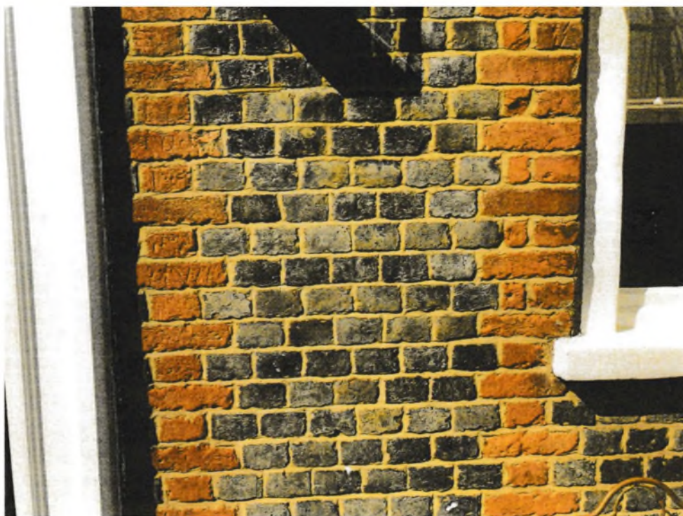
Fig.2 Detail of no. 33 West Street showing the use of the prevailing blue brick in Header Bond with red brick edging the window frames.
