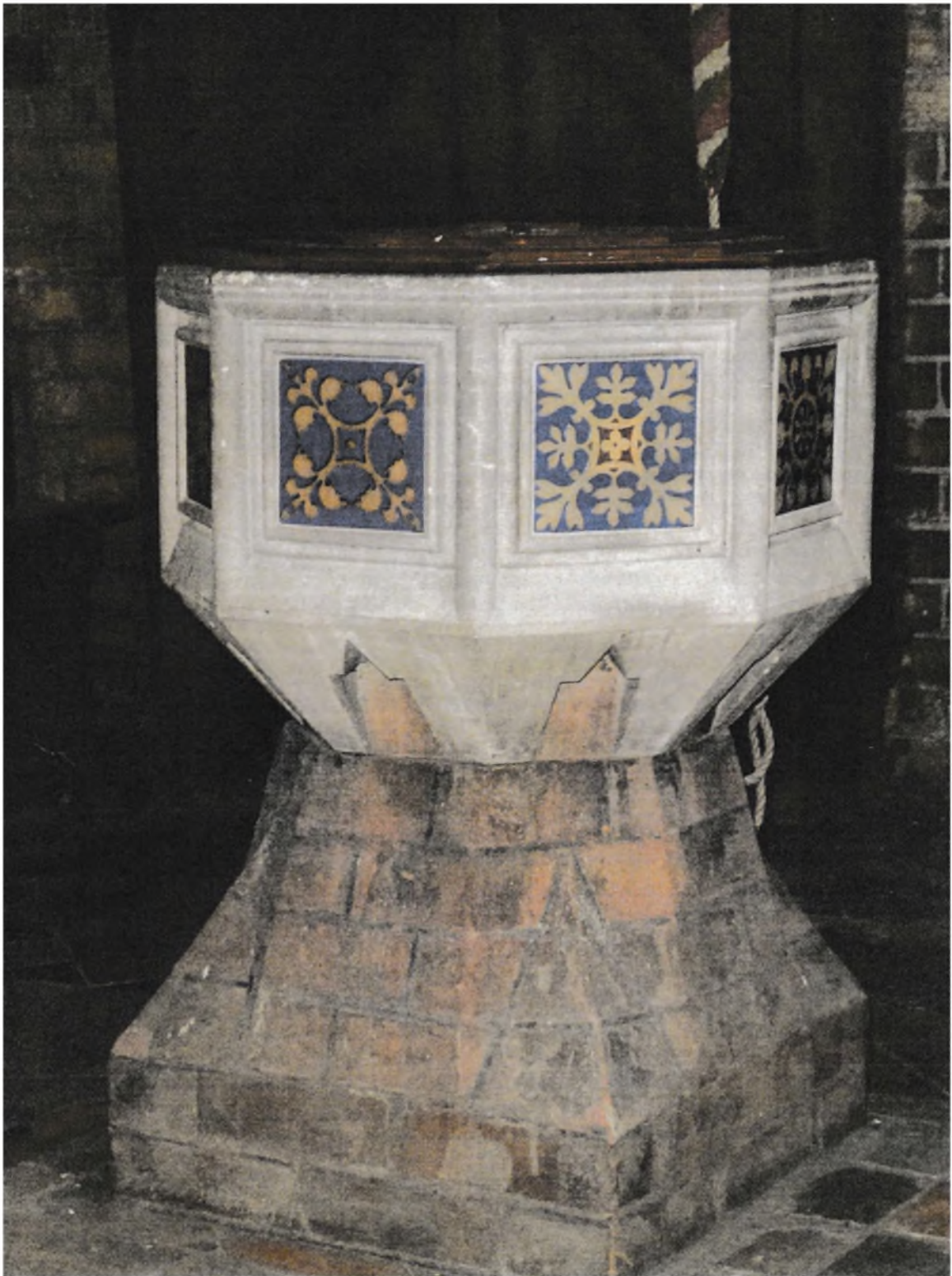
Fig.10 Burringham church: the font with brick base and blue and cream encaustic tiles set into the octagonal stone bowl.
