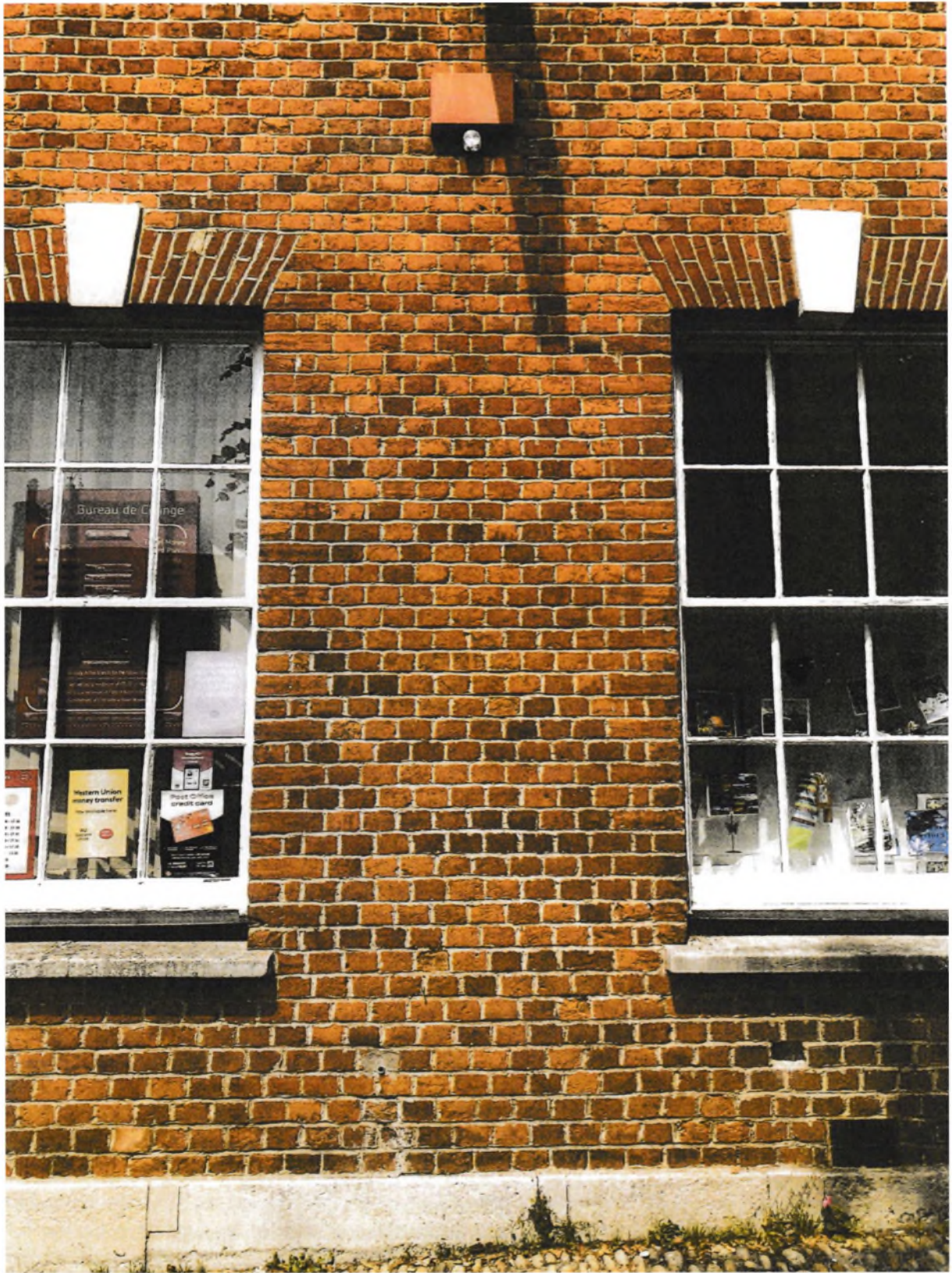
Fig.4 Greville House, West Street, Bridport, now the town's Post Office, is a house built in red brick laid in Header Bond.
