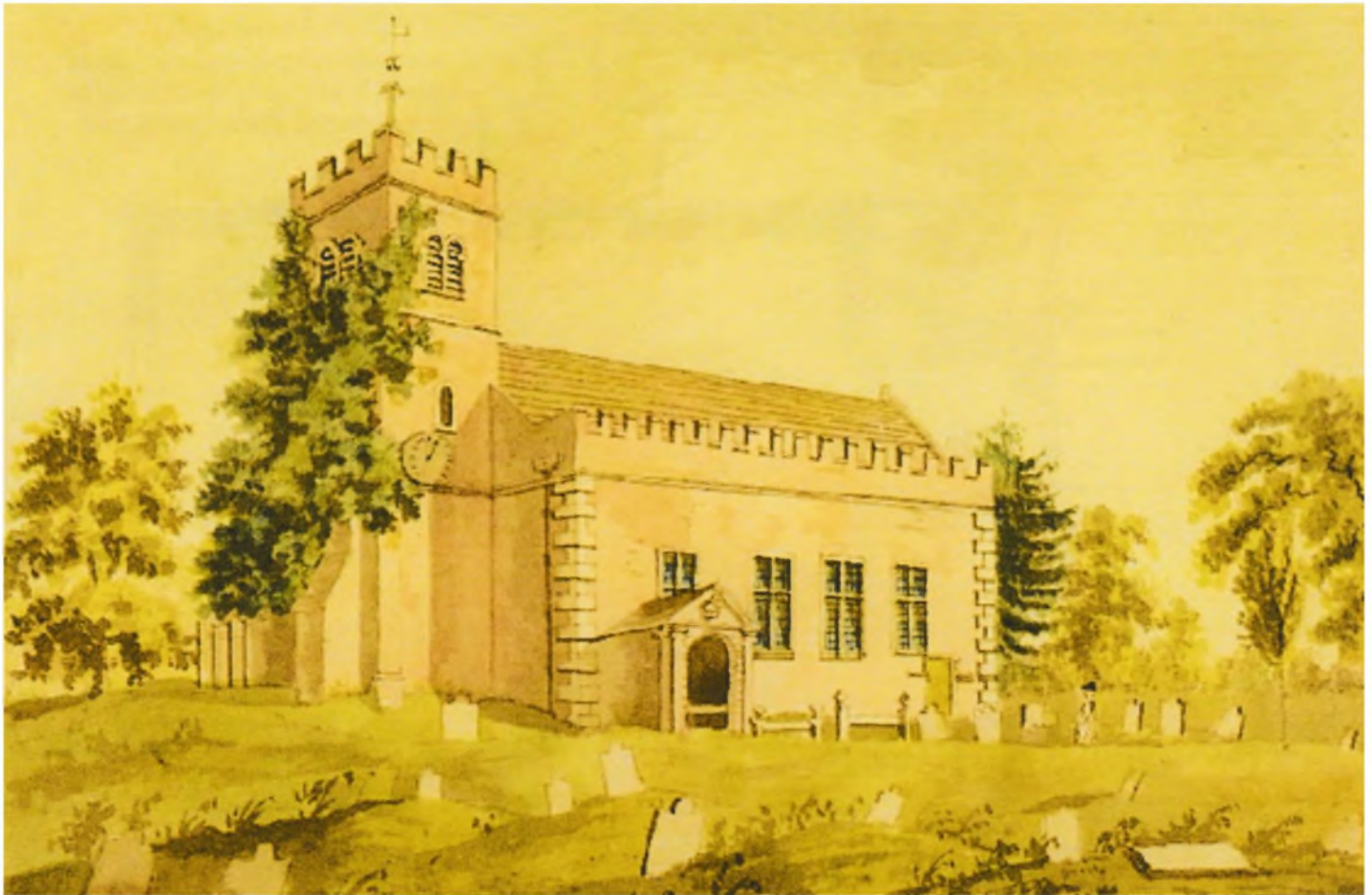
Fig.4 A painting of the south side of the church made circa 1800. This shows the porch of Portland stone carved by Nicholas Stone and the four windows with wooden frames for the glass consisting of a single transom and a single mullion. There is a small door at the east end. Note also the presence of the supplementary buttresses to the west side of the west tower.
