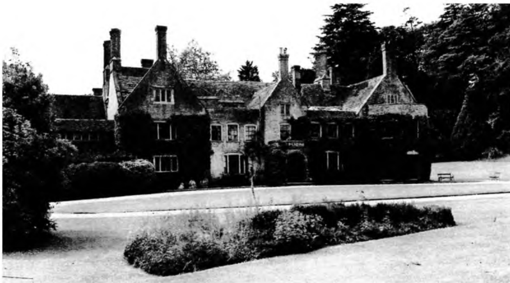
Fig.6 Bloxworth House, a double pile house of 1608 with an E-plan front in red brick with two rows of stretchers to a single course of headers.
