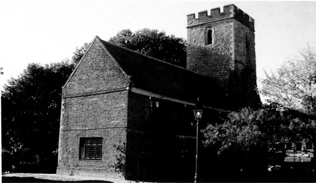
Fig.1 The Plume Library, Maldon, Essex, on the site of St Peter's church: the two easternmost bays were built in 1817, with a window only to the ground floor. The building retains the church's fifteenth-century west tower of flint.
