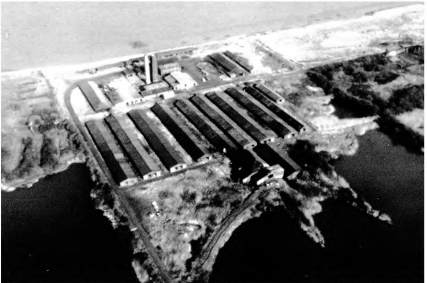
Fig.2 Aerial view from south-west of Blyth's Hill brick and tile yard, 1976. The River Humber is at the top of the photograph; flooded clay pits at the bottom. The components of the yard and their layout are typical of the larger brick and tile yards in the Humber estuary. Ken Redmore collection.
