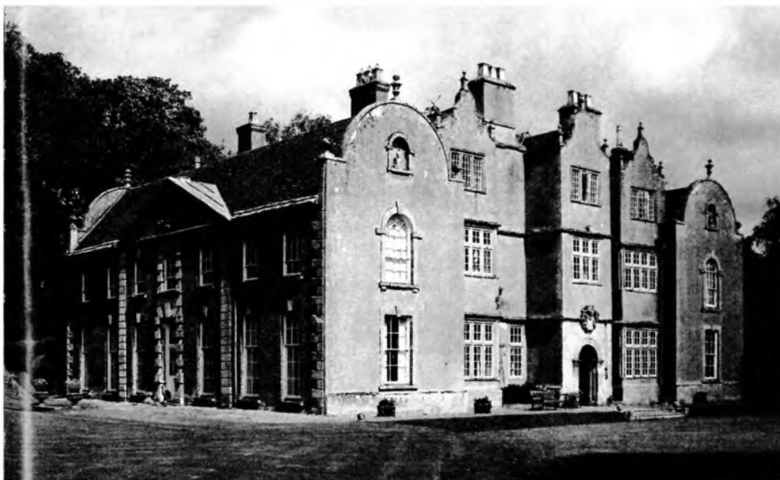
Fig.5 Edmondsham House: the central five bays are the late-sixteenth-century house with an E-plan front, the single outer bays are eighteenth-century replacements for the original wings.
