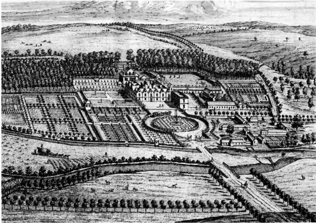
Fig.3 Bryanston House in the first decade of the eighteenth century, the late-sixteenth-century courtyard house with a set of six gables on the front. By 1707, there were two additions: a banqueting house of circa 1640 with a flat roof at the front of the house and a large building with a hipped roof at the rear, built circa 1685. The parish church is to the right of the banqueting house with agricultural buildings to both its east and west. Engraving from Thomas Kip, Britannia Illustrata , 1707, plate 97.
