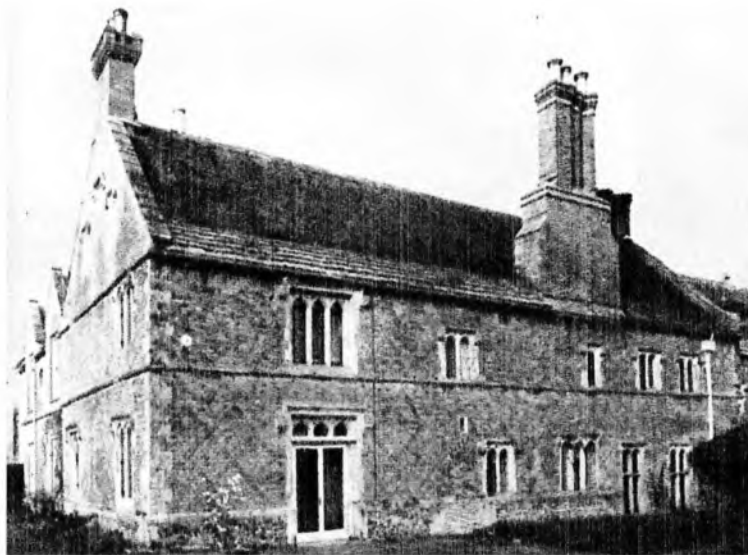
Fig.2 Abbey House, Witchampton: the early-sixteenth-century wing, of red brick with over-fired headers as diaper.
