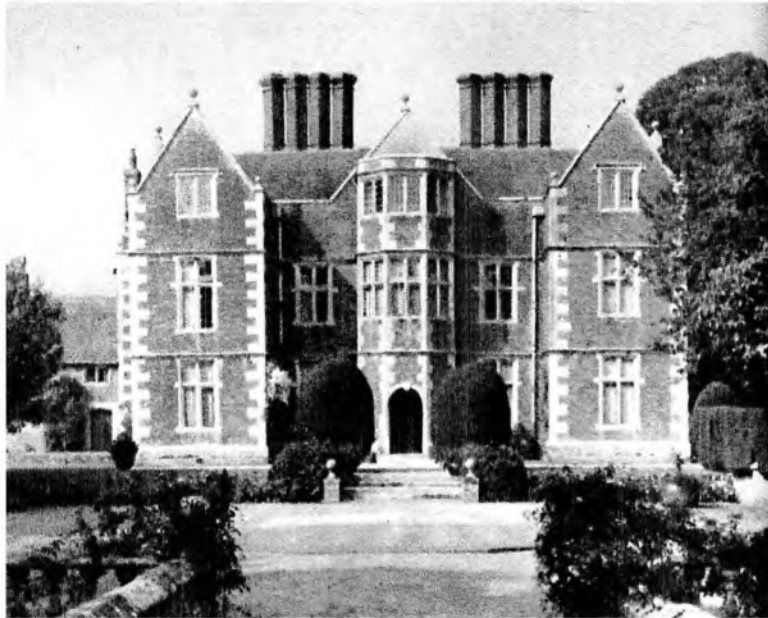
Fig.7 Anderson Manor, a house built in 1635 with an E-plan front where two rows of stretchers in red-brown brick alternate with a single row of headers in grey brick. Note the chimney stacks along the spine of the double pile house as the feature of the recessed bays.
