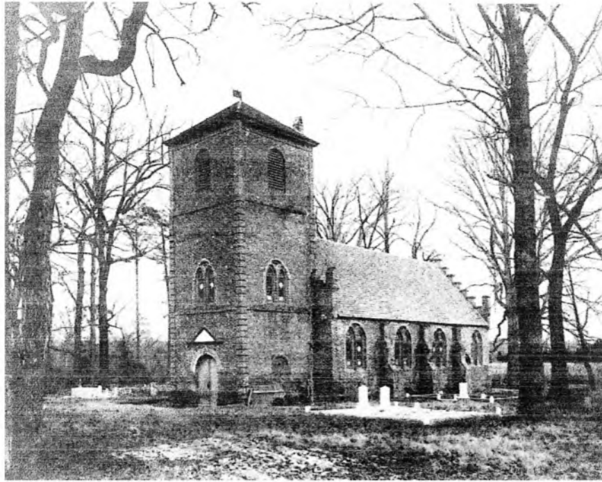
Fig.3 St Luke's church from the south west, circa 1865, showing repairs around the windows and the prominent buttresses. (Photograph after Dell Upton, Holy Things and Profane , New Haven and London: Yale University Press.)
