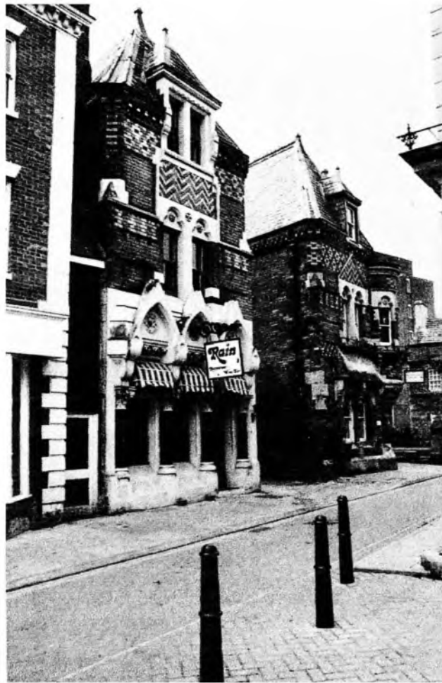
Fig.3 Nos. 24 and 25 Cornhill, in polychrome brickwork: no. 24 was a shop, but no.25 was a private house. Both were erected as eyecatchers for the owner of the nearby Castle House, W.J. Douglas.
