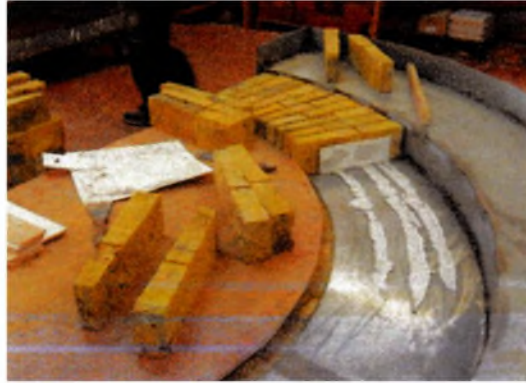
Fig.2 (right) Reclaimed London Stock bricks being arranged on a semi-circular, stainless-steel former to create the beginnings of an arch.
