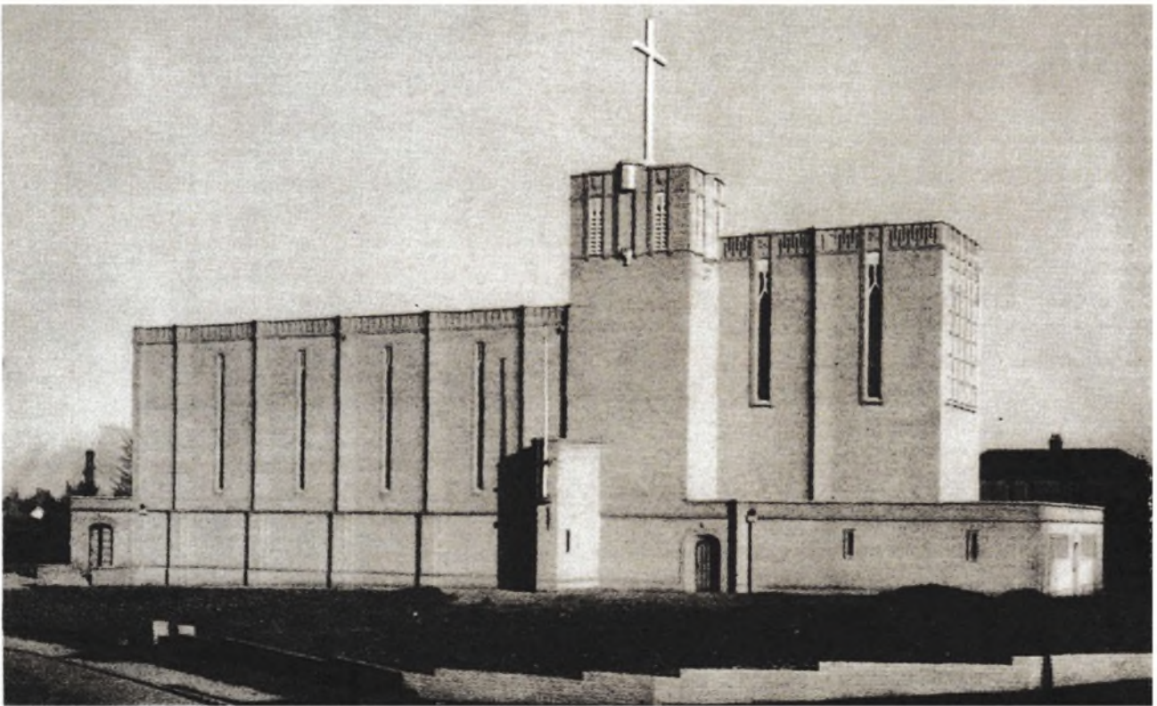
Fig.10 (top) St Barnabas, Tuffley, Gloucester (1939-40: N.F. Cachemaille-Day): interior showing concrete ribs supporting the roof. Fig.11 (below) St Barnabas, Tuffley: exterior from the south with tower at junction of nave and chancel, which houses the organ pipes.
