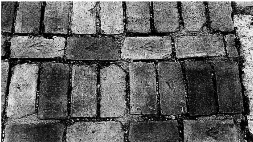
Fig.1 Bricks re-used to make steps for visitors.
