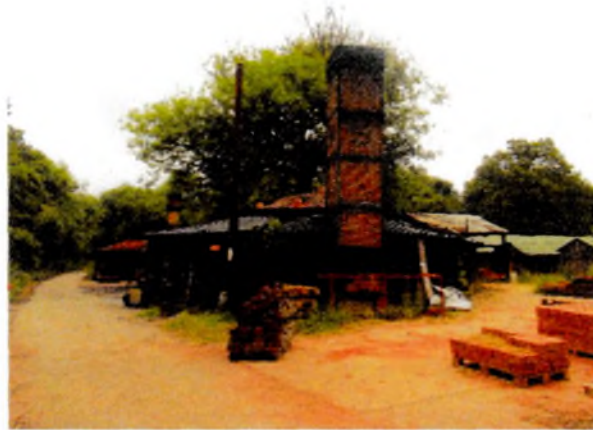
Fig. 17 View of both the kilns, with a chimney stack providing the ‘draught’ to circulate the hot gases through the setting to raise the temperature and to remove the unwanted products of combustion.
