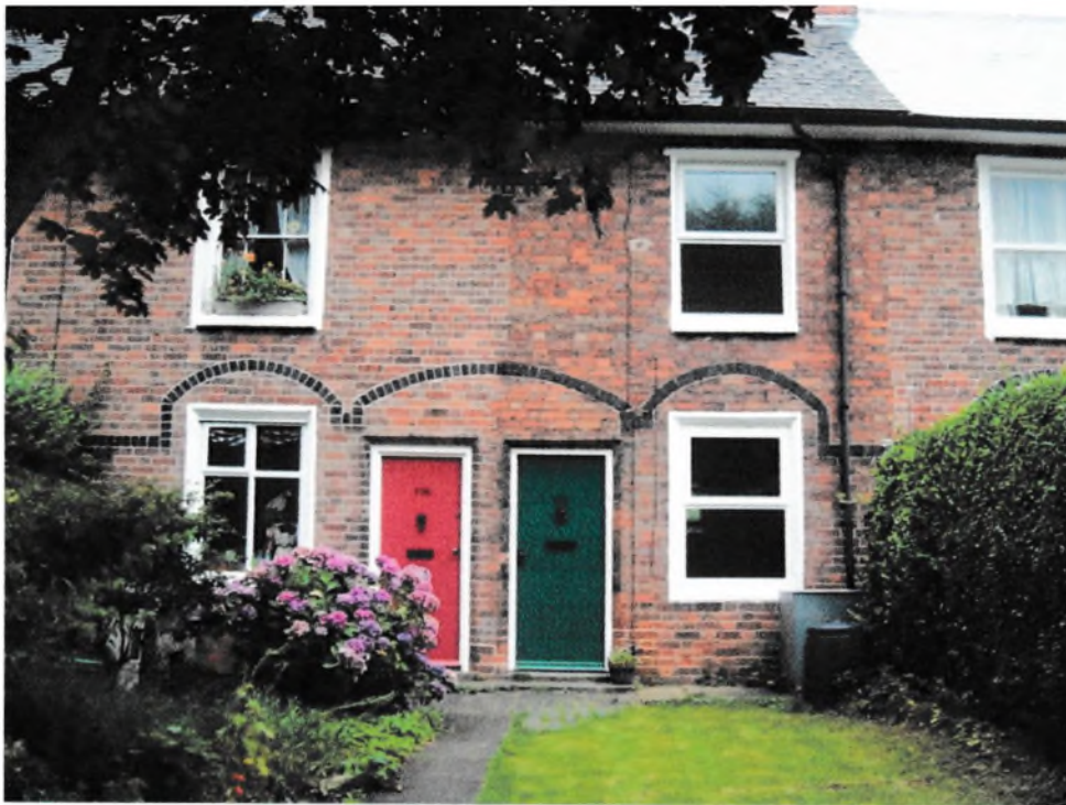
Fig.5 Fern Cottages Woodborough Rd, Nottingham. The distinctive blue brick string course would have involved an extreme amount of work for the bricklayers, bricks having to be cut to size above and below the arching. A sure sign an architect was involved with the project!
