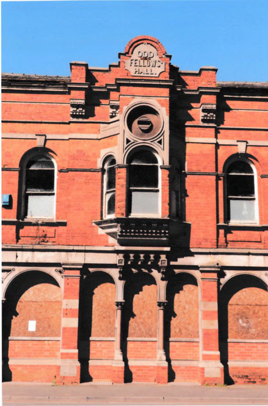
Fig.11 (left) The central portion of the Odd Fellows Hall, Unity Square, Lincoln, with architectural fittings by Fambrini & Daniels.
