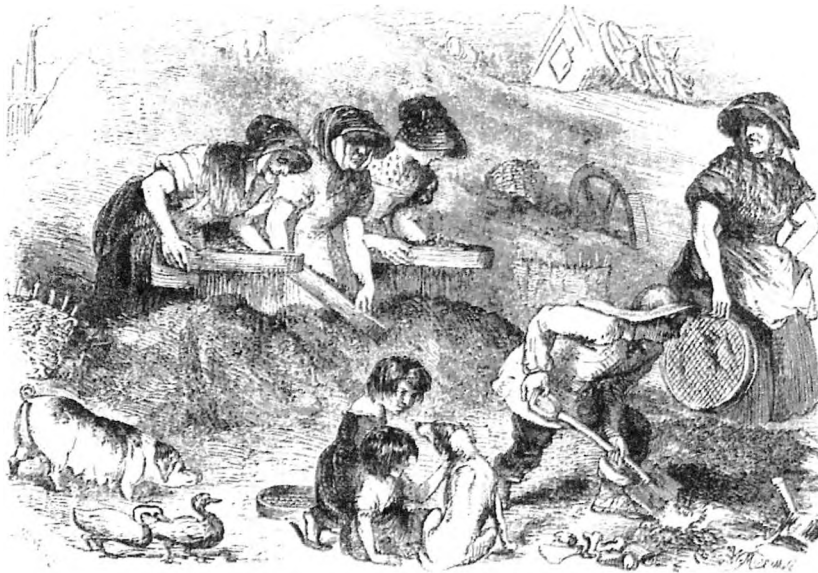
VIEW OF A DUST YARD. (From a Sketch taken on the spot.)
