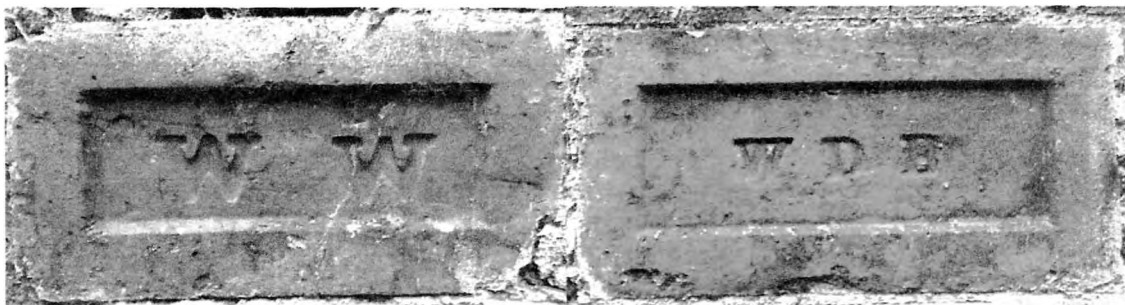
Fig.1 Bricks from the wall alongside the entrance road to the Greenfoot public car park, Settle, North Yorkshire, with the marks WW and WDB. Photograph: Mike Chapman
