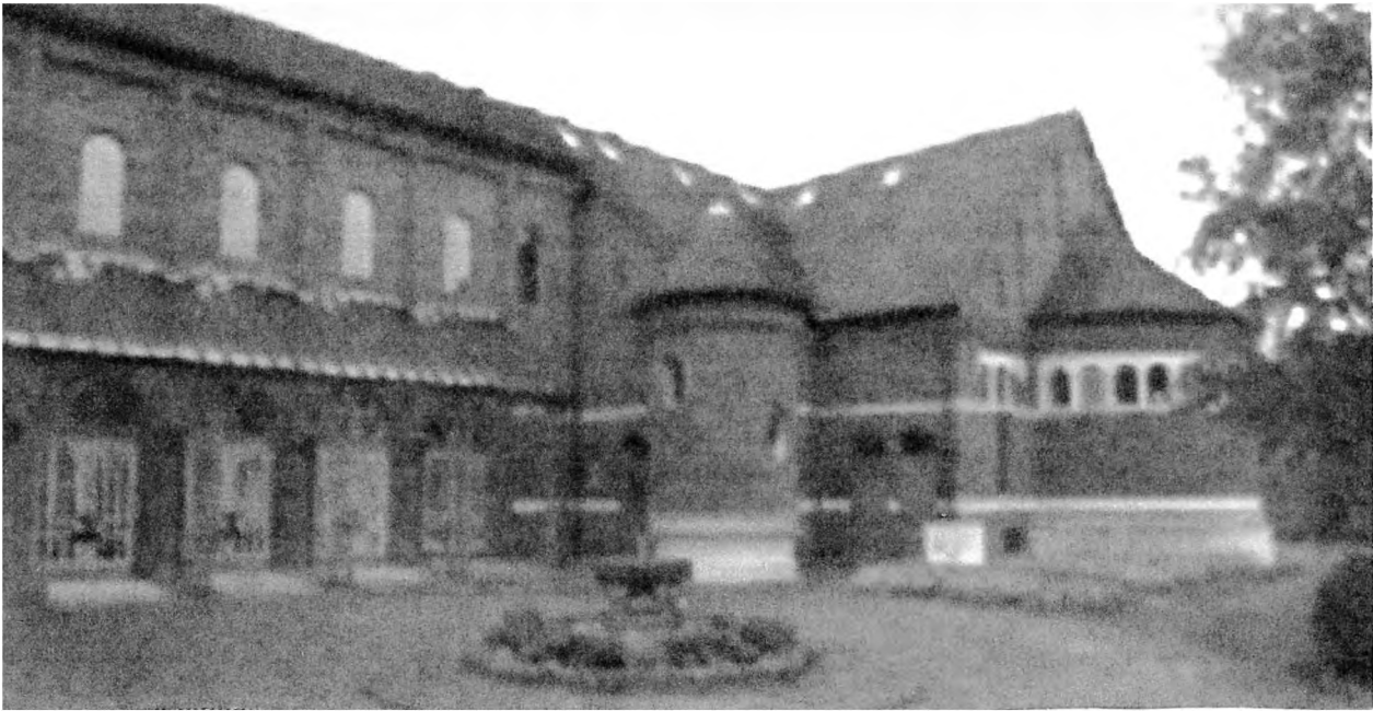
Fig.4 St Francis of Assisi church, Kenilworth, Warwickshire (1992-93: Rathbone & Taylor), a relatively conventional cruciform design but with the south transept given an extension in the form of a quadrant of a circle to accommodate a raised baptistry, allowing the priest and the family to stand behind and to the side of the font in comfort and the congregation to be witness to the christening. The building is clad in red brick laid in a mixture of bonds, including Header Bond in the curved areas. The long narthex connects with the social spaces beyond.
