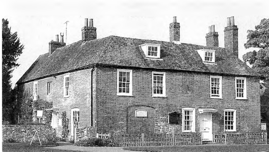
Fig.3 Chawton Cottage, Chawton, Hampshire, a timber-framed building modernised by using brick tiles (mathematical tiles) to up-date its appearance. This was the home of the novelist Jane Austen (1775-1817), her sister Cassandra and her widowed mother from 1809.
