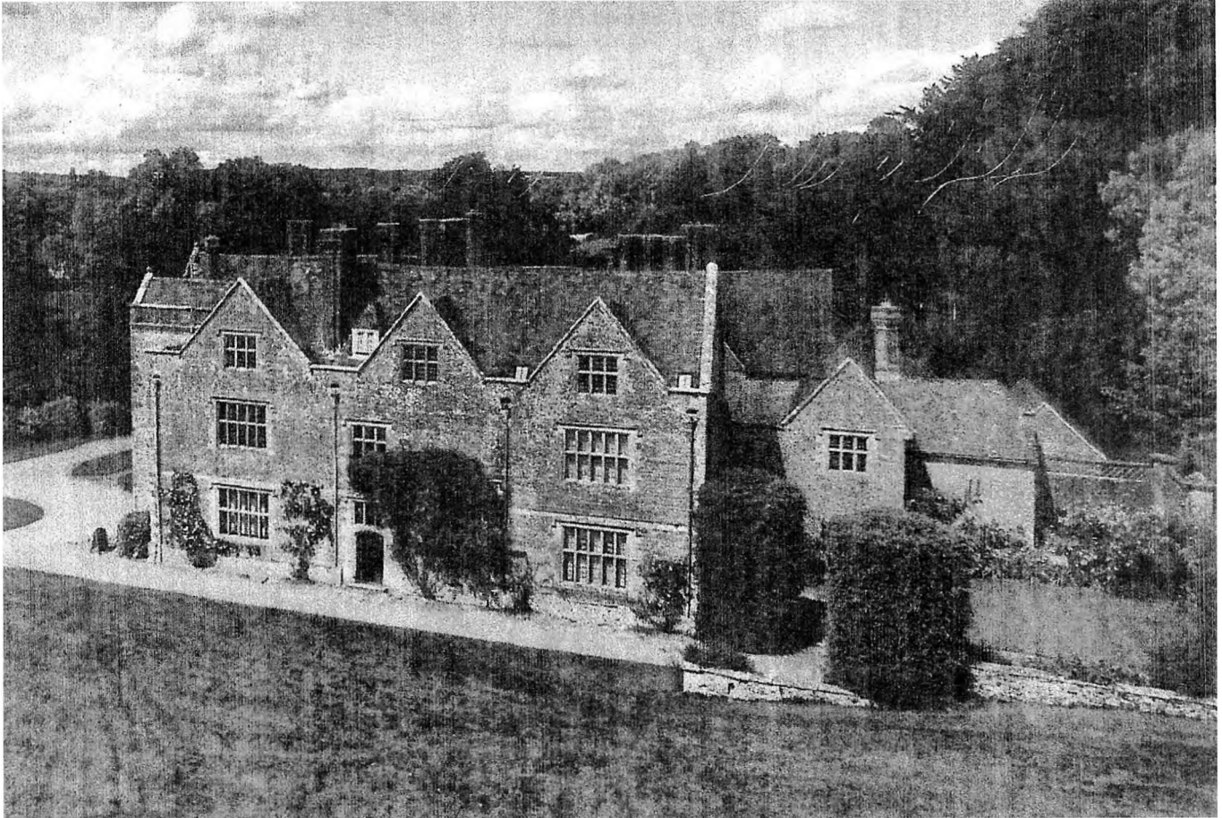
Fig.2 The original, E-plan south front of Chawton House, Hampshire, with three gables built for Richard Knight in 1583. The mainly brick structure has stone dressings and stone mullions and transoms for the windows. Within a decade, the internal arrangements had been re-ordered and a west front had been built of Hampshire marlstone.
