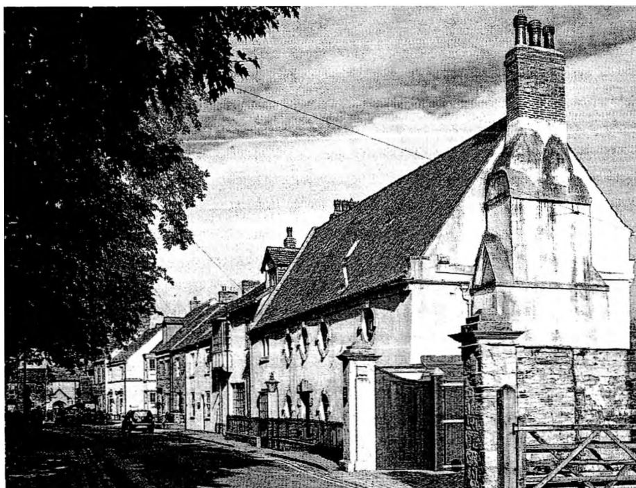
Fig.2 The north front of St Agnes Lodge, Ripon, North Yorkshire, showing the steep pitch of the roof, the large chimney stack of with arched decoration rebuilt circa 1700 on the right, and on the left, windows of the easternmost bay, replacing a mid-Victorian Gothic-style bay window. The oculi of the other four bays were installed in the 1730s or 1740s. The render is recent and lime-based.
