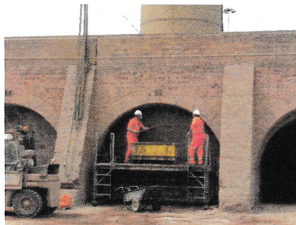
Fig.18 Bricking up and sealing the kiln entrance, or wicket, once the chamber has been filled.
