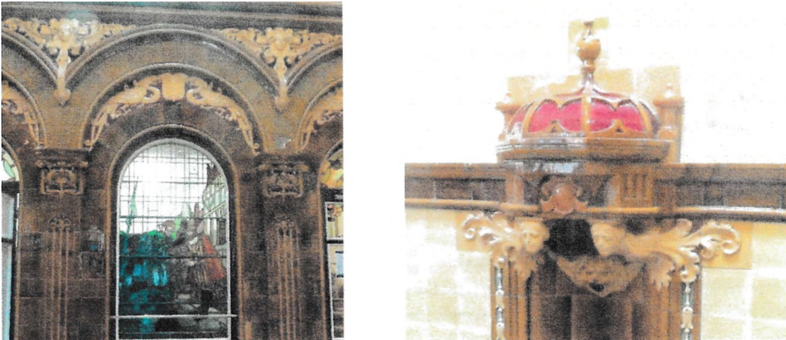
Fig. 2 (right) Faience ware at the Bath Spa, Ripon, by Burmantofts of Leeds.
