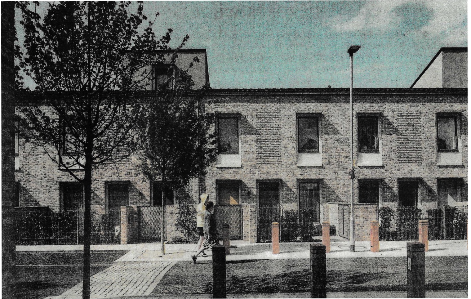
Fig.1 Goldsmith Street, Norwich: new two storey, brick-built houses on a mixed development of family homes with three-storey flats. Every dwelling has a street door facing its neighbours and without cars blocking the street.
