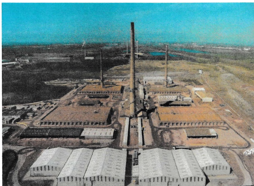
Fig.1 Aerial View of Forterra's Kings Dyke Works, Whittlesea, Cambridgeshire.
