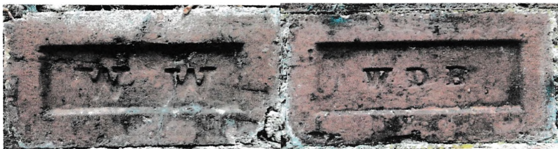
Fig.2 Bricks from the wall alongside the entrance road to the Greenfoot public car park, Settle, North Yorkshire, with the marks WW and WDB.
