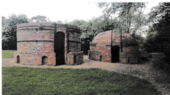
Fig.1 The two beehive kilns at Great Linford showing the entry point for loading and unloading.
