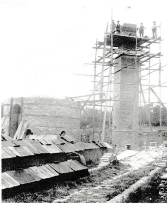
Fig. 3 Photograph showing the construction of the chimney and newly completed kiln which clearly show the iron "buckstays" on each side of the wicket entrance and the hoops that kept the kiln together during the expansion and contraction of intermittent firing.
