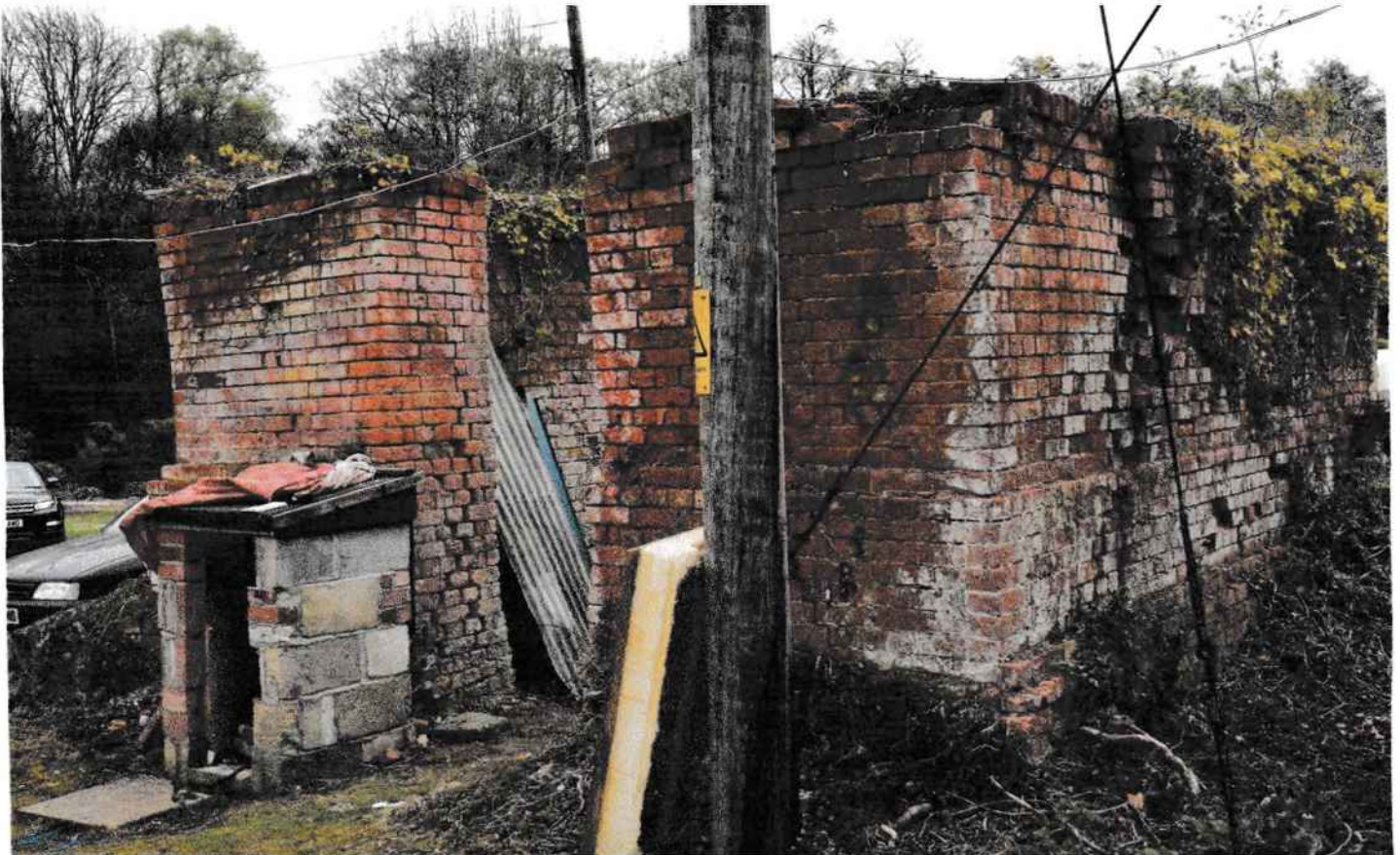
Fig.5 Remains of a scotch kiln just outside Chandlers Ford (now demolished). Dating from around 1900 it is thought to be similar to many of the kilns used on The Main Site.
