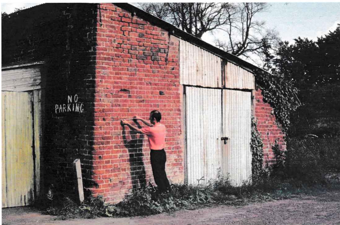
Fig. 9. Tony Ward, a founder member of SIAS and leader of the project to survey Hoffmann Kiln No.2 at Poole Works, Wellington, examines the Blue Anchor kiln bricks for texture, colour and dimensions. One eye or grate is at ground level on the left. Image courtesy Brian Murless
