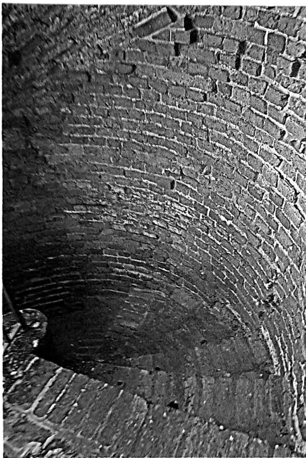
Fig.2 Kirby Muxloe Castle, 1480-83. One of the four brick staircases in the castle. The vault is seen at the top left-hand. (Jeremy Polanski, Flickr, Creative Commons Licence)
