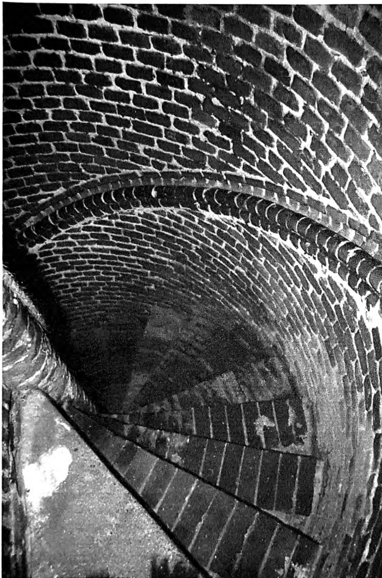
Fig.5 Rye House, Hertfordshire, 1443. The handhold is particularly fine. The newer darker bricks to the treads are replacement Staffordshire blues and the tread in left foreground is faced up with sand and cement. (M. Tutton)
