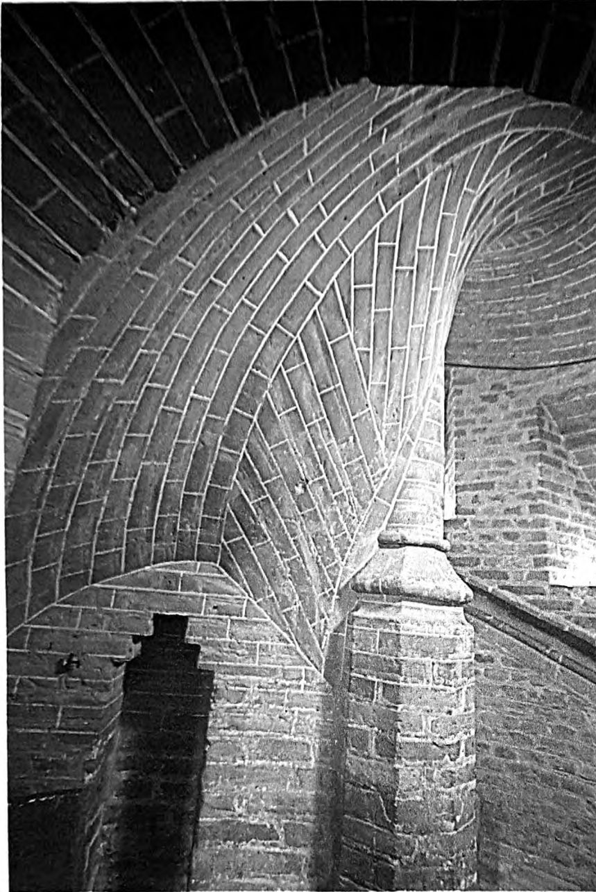
Fig.3 Oxburgh Hall, Norfolk, c.1482. Bottom of the staircase with the base of the newel, lamp niche and handhold. Note the lining out of the pointing to the underside of the vault. (M. Tutton)
