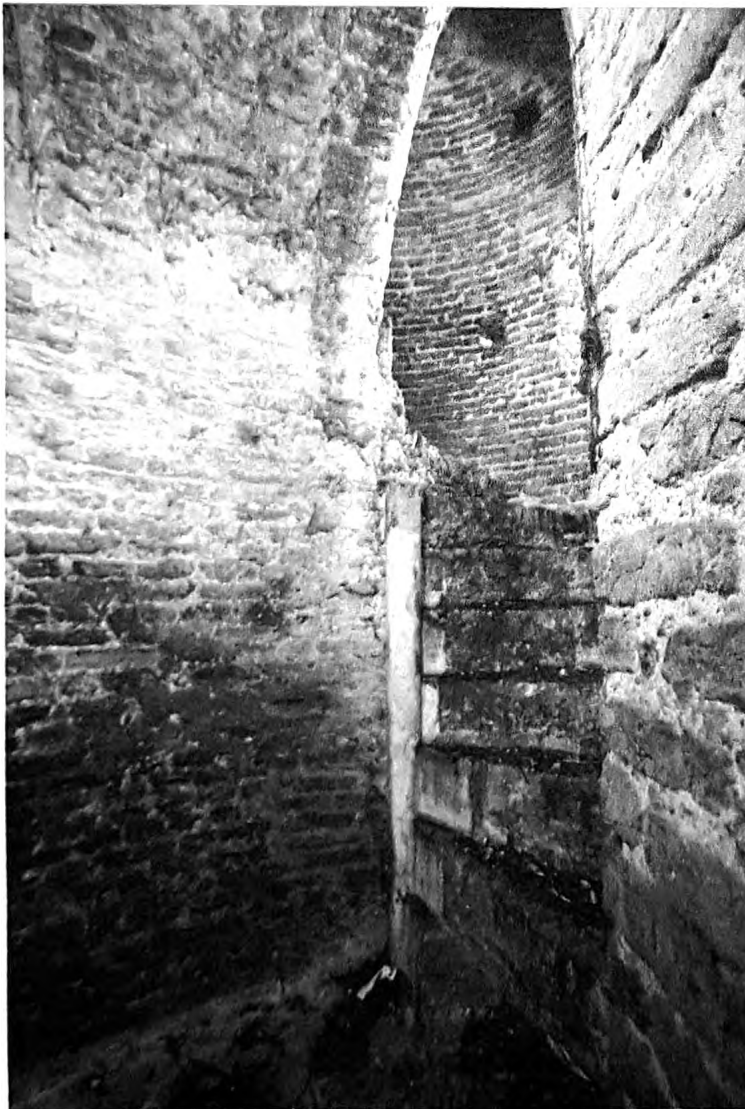
Fig.1 Cow Tower, Norwich, 1398. Brick stair with stone newel. Note the arch radiating from just above the dark hole or putlog in the upper right-hand. (M. Tutton)
