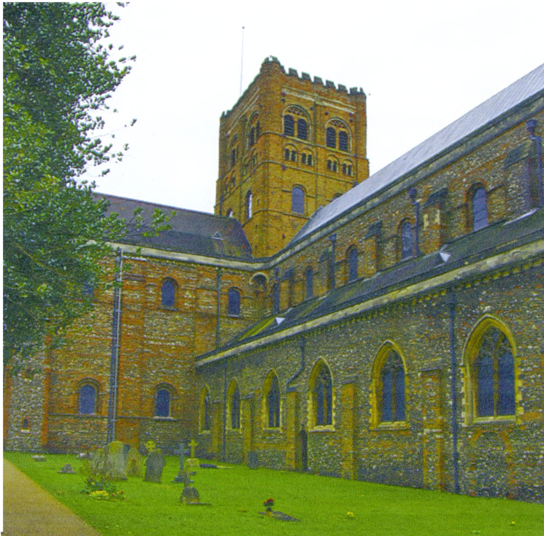
Fig.3 St Albans Abbey: the north side of the nave and the west side of the north transept are mainly built from reused Roman bricks, sourced from the Roman town of Verulamium.
