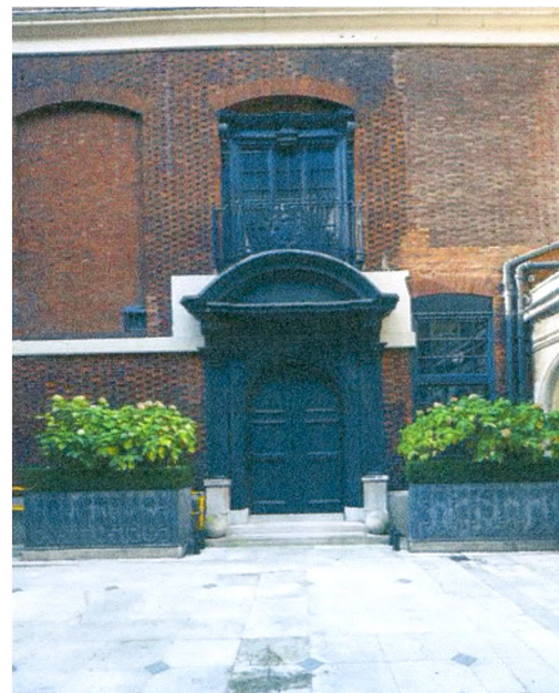
Fig.1 (left) The wall of the hall of the Skinners' Company, City of London, with diagonal striations on both the stretcher face of the orange-brown bricks and the header face of the black bricks.
