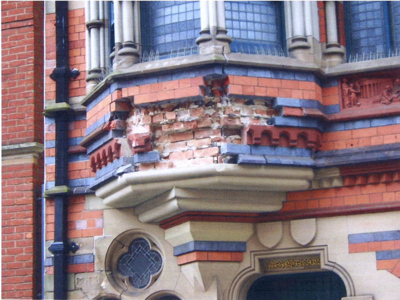
Fig.3 The damage to the oriel window. Externally, in the oriel window above the stone plinth are a course of 45° angled Staffordshire blue bricks, a course of Staffordshire blue bricks, a course of specials in deep red being the height of two courses, a course of Staffordshire blue bricks, a course of deep red 45° angled bricks, a course of Staffordshire blue bricks, two courses of red facing bricks, a course of Staffordshire blue bricks, and the stone sill below the windows.
