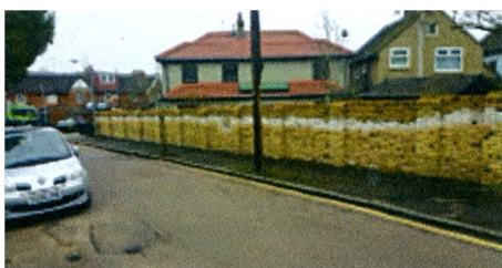
Fig1 (right) General view of the garden wall with efflorescence.
