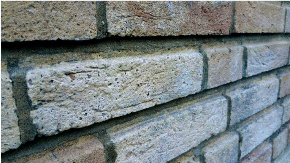
Fig.2 The illusion is achieved by using the rebated bricks with flush pointing of the vertical joints; view looking along the joints.
