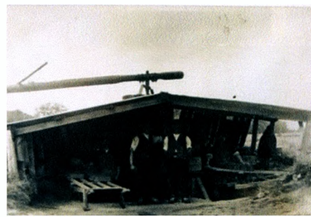
Fig.4 (right) Horse-drawn pug mill for hand-made brickmaking with bearing-off barrow for transporting the green bricks to the drying hacks.
