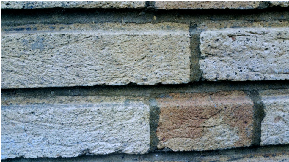
Fig.3 The rebated bricks, a view looking directly at the brickwork.
