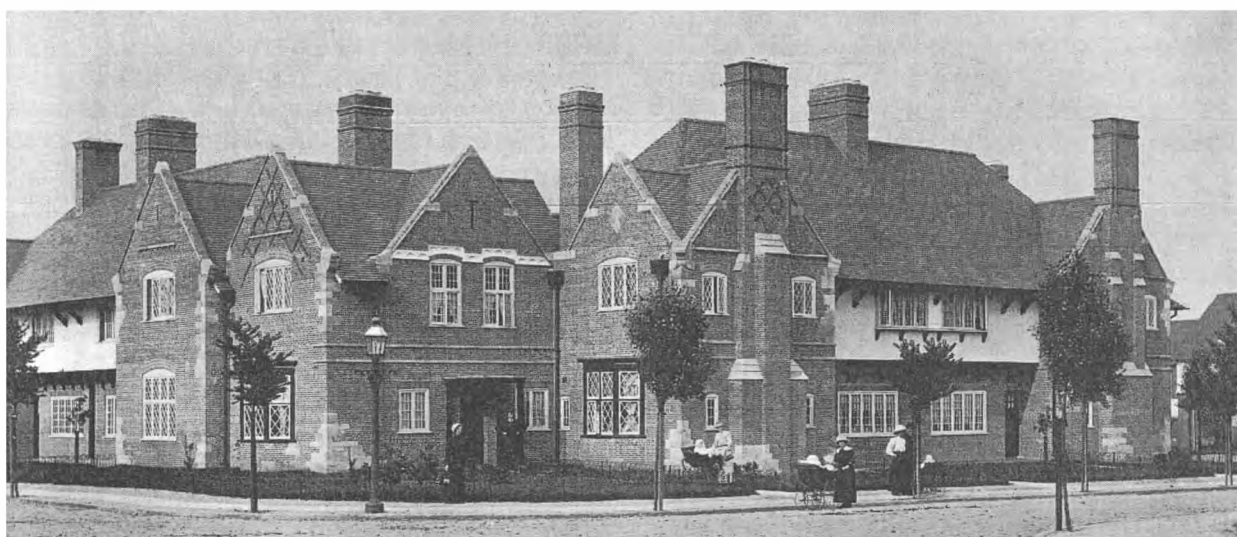
Fig.6 Co-joined houses at the junction of The Causeway and The Diamond in the centre of the post-1912 formal layout adopted for the main thoroughfare of the village. These houses by James Lomax Simpson feature much use of black diaper in the mainly red brick façades.
