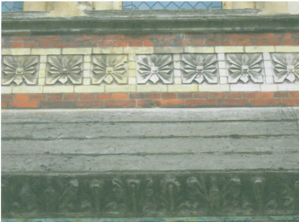
Fig.6 Close up of Pether's Patent Bricks as used below the west window of St Augustine's church, Queen's Gate, South Kensington.
