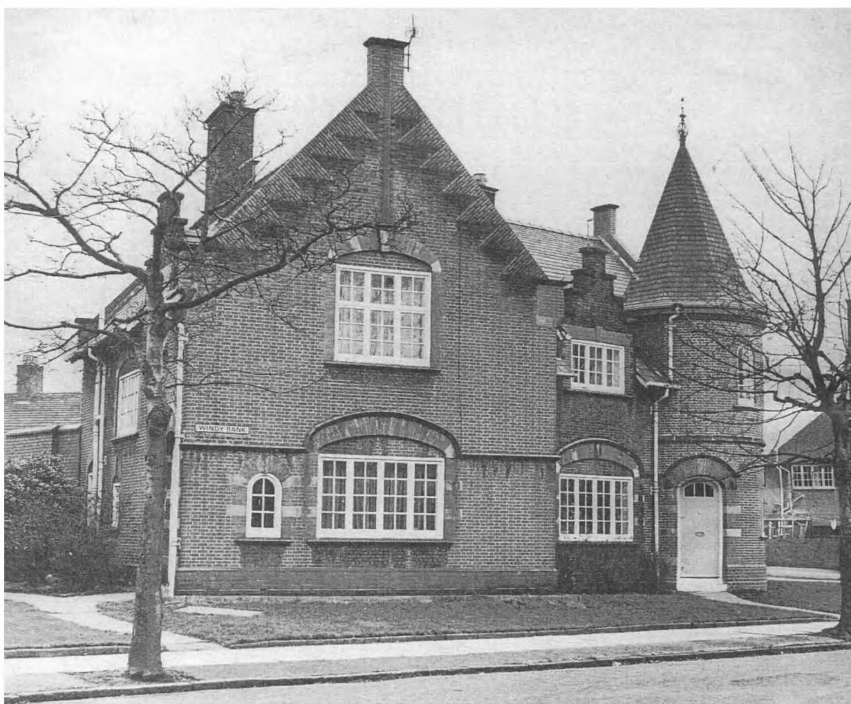
Fig.5 The 'Belgian Cottages' at 23 and 24 Windy Bank, were built of bricks imported from Belgium and feature tumbling in a high gable and crow-stepped gables.
