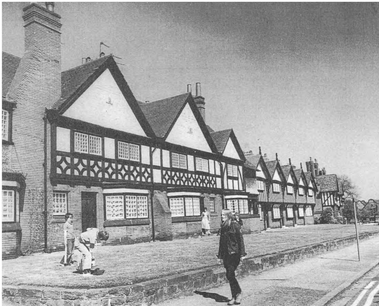
Fig.2 Two early blocks designed by William Owen, numbers 1-7 and 9-17 Park Road, with the ground floors and chimneys of red Ruabon brick but timber-framing on the first floor. The two houses on the left have pargetting in the gables with 'LBL' in one and '1892' in the other. The houses at the end of Park Road were designed by D.P. Fordham of Douglas & Fordham and unusually have roofs of stone slates.
