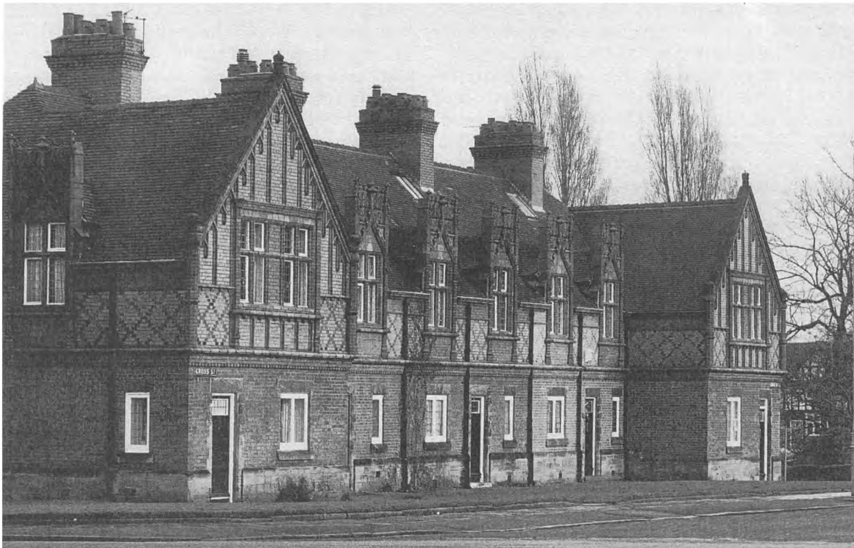
Fig.3 Five houses on Cross Street, built in 1896 to designs by Grayon & Ould of Chester, have elaborate diapered brickwork on the first floor and terracotta in the gables to the dormer windows.
