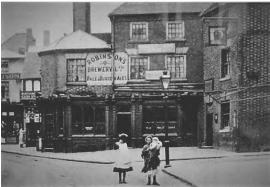
Fig.3 Early-twentieth-century photograph of central Bedworth showing chequered brickwork prominently on the gable wall of the public house and less easily discerned on the wall with the brewery sign. Light-coloured headers and darker stretchers can be seen below the wall advertisement.
