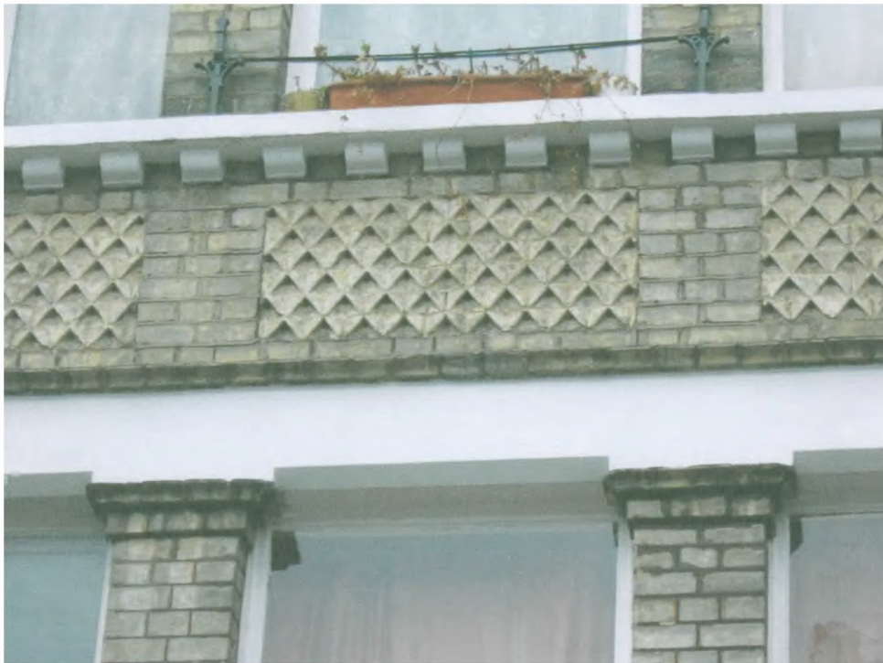
Fig.2 Pether's Patent Bricks in three panels below the second-floor windows of 9 Kenway Road.
