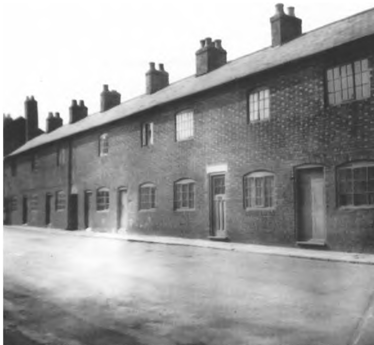
Fig.1 Cottages in Bedworth, Warwickshire, built in Flemish Bond using light-coloured headers and red stretchers, probably erected in the early nineteenth century in date
