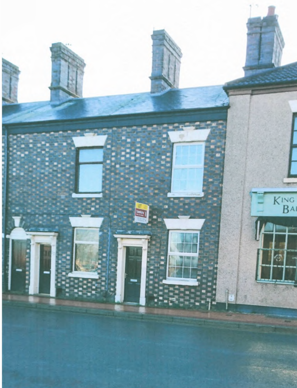
Fig.2 Late-nineteenth-century terraced houses, King Street, Bedworth, Warwickshire, showing very dark stretchers laid with light headers.
