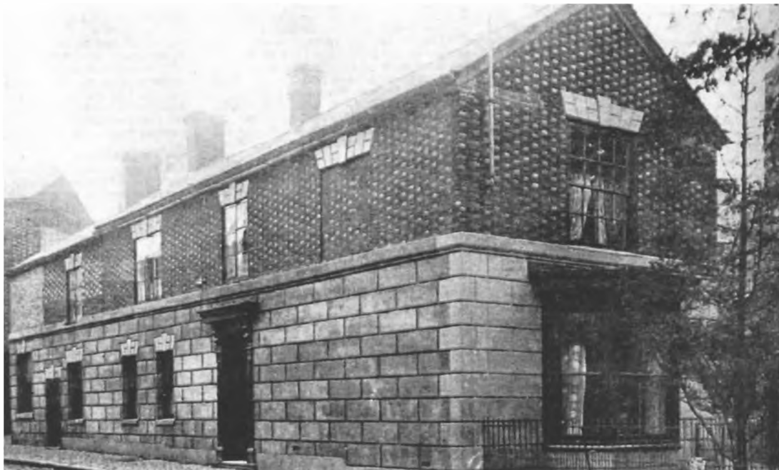
Fig.6 Congreve Hall, Market Place, Bedworth, with the first floor and end gable in chequered brickwork of light-coloured headers and darker stretchers.
