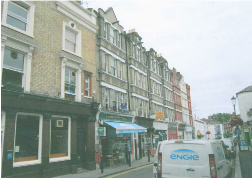
Fig. 1 Prince of Teck Buildings, 1-13 (odd numbers) Kenway Road, Earl's Court, London SW5, completed 1881: general view from south-east with Pether's Patent Bricks used under the windows of the second and third floors. The shaped gable has been removed from number 1 and replaced on number 13. The protruding bar is to enable a hoist to be used to allow furniture to be delivered to rooms on the first, second, and third floors.
