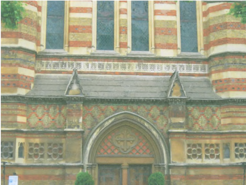
Fig.5 St Augustine's church, Queen's Gate, South Kensington, close up of Pether's Patent Bricks on the west front.
