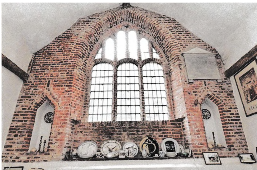
Fig.3 The former All Saints church, Langdon Hills, Basildon, Essex: the brick tracery of the sixteenth-century east window from the interior. Note the presence of niches for statues, a pre-Reformation building practice. Both this photograph and that reproduced as figure 2 show that the base of the window has been raised.
