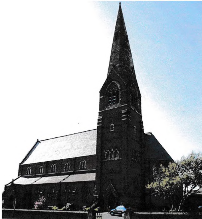
Fig.2 St James, Barrow-in-Furness, designed in 1867 and completed in 1869 has a wide nave with clerestory, aisles, a polygonal apse, and an asymmetrically-placed south-east tower capped by a spire. The red brick interior was originally matched by an unplastered interior; today the red brick arches of the six-bay arcades and the chancel arch contrast with the plain white of the rest of the church.
