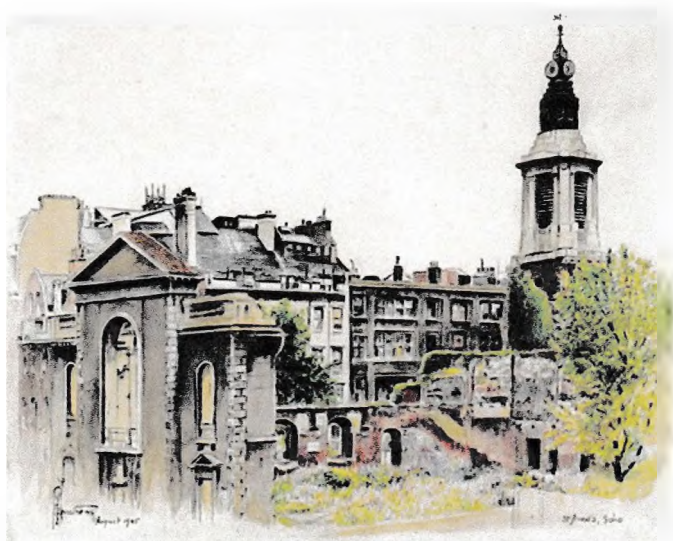
Fig.1 Painting of St Anne's church, Soho, in August 1945 by R.G. Matthews. This shows the extent of the bomb damage and also the internal red bricks. In the final century of its life, the exterior of the seventeenth-century church and its eighteenth-century tower were covered with stucco although the stone quoins of the east end were left proud.
