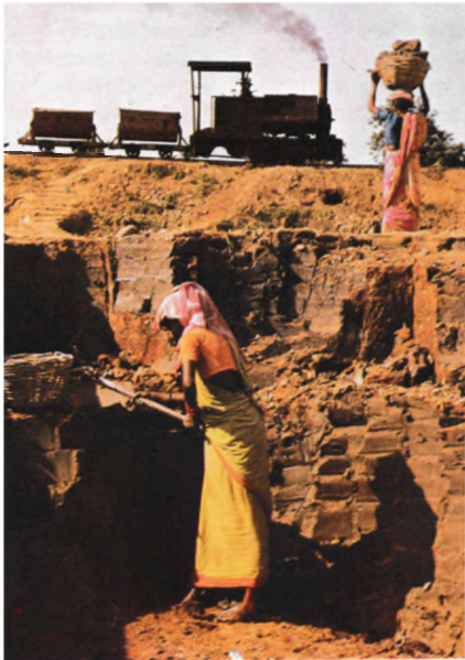
Fig. 1 (left) Gaily-dressed women hack brickmaking clay from the claypit servicing the British-built brick kilns at Ledo, in north-east Assam, India. Other women carry the brick-sized and brick-shaped clay lumps to the waiting transport. The clay is taken on a narrow-gauge railway in tipper trucks to the brick kilns. A photograph from the 1970s.
