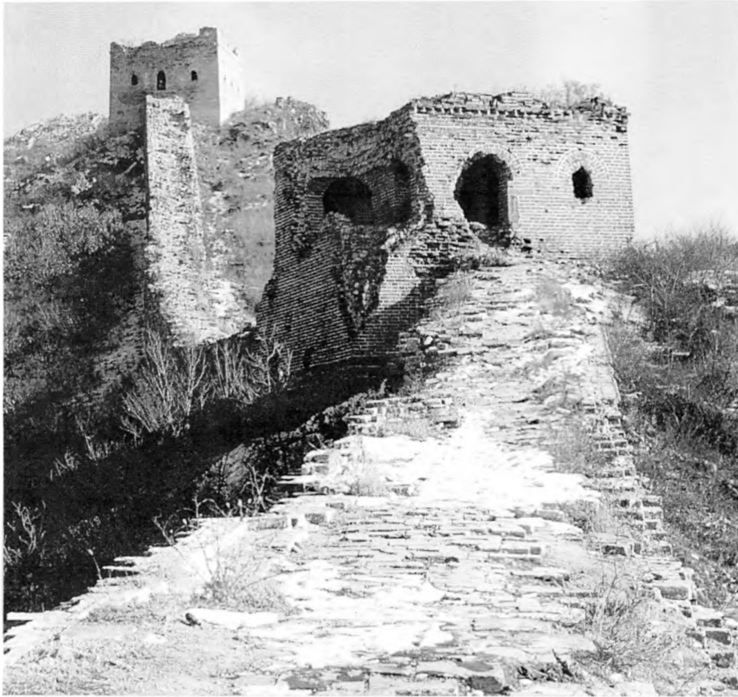
Fig.2 Throughout its length, the Great Wall of China has watchtowers at regular intervals. This photograph of the brick built wall in north-east China shows two ruined towers, one at a much higher elevation than the other. Both, however, sit on the edge of a precipitous cliff. The wall, here in a partly ruinous state, is set back from the edge of the cliff. Originally, there would have been parapets both at the front and the back of the brick-floored walkway.
