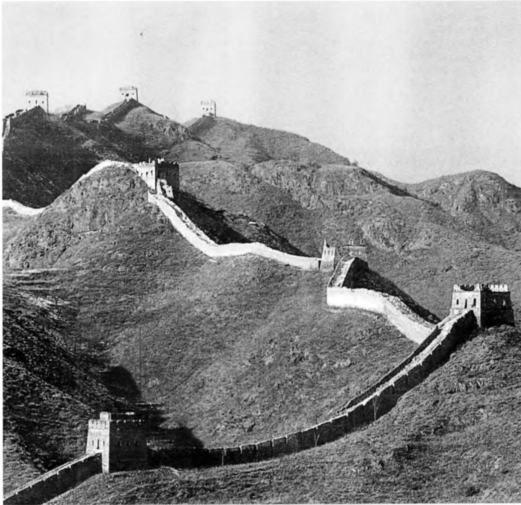
Fig.1 The Great Wall of China commands the high ground and takes no account of the local topography. Here the brick-built wall and the regular watchtowers snake across the landscape of north-east China north of Beijing. The parapet is clearly visible.
