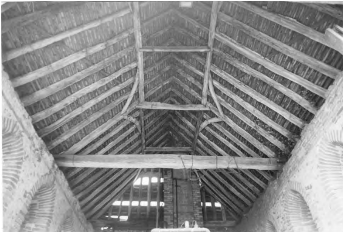
Fig.3 Little Coggeshall Abbey, the roof of the abbey guesthouse. Note the brick arches of the lancets with above them three courses of brick added in the sixteenth century when the present roof was installed.
