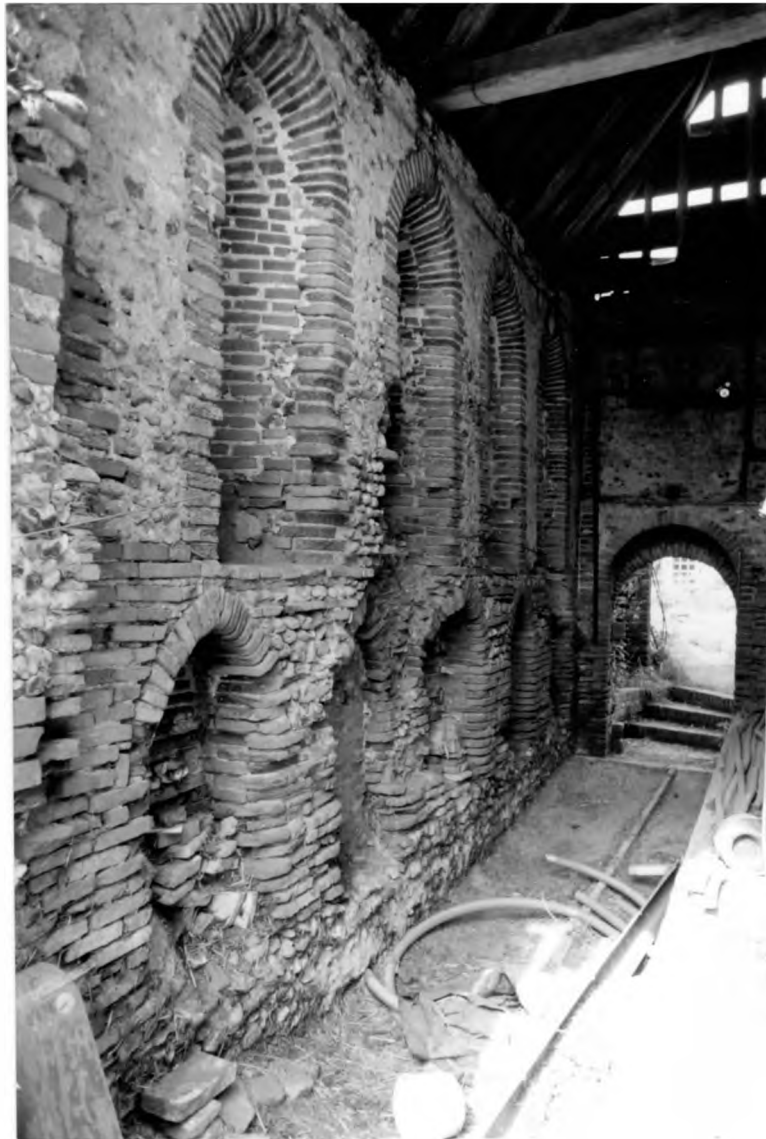
Fig.2 Little Coggleshall Abbey, internal view of the west wall of the abbey guesthouse showing relieving arches on the ground floor and lancets on the first floor. The round-headed doorway in the north wall is original. The return on the extreme left of the photograph is the scant remains of the south wall of the guesthouse.
