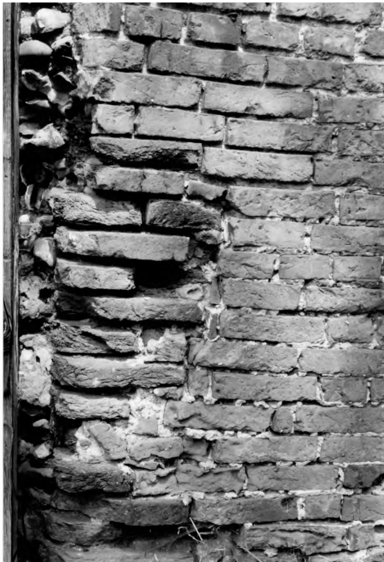
Fig.1 Little Coggeshall Abbey, external brickwork at the abbey guesthouse, built circa 1190.
