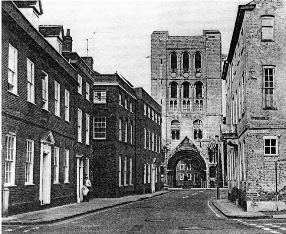
Fig.2 Houses on the left-hand side of Churchgate Street were built in red brick, sometimes over an earlier, timber-framed house; those on the right-hand side were built in yellow brick.
