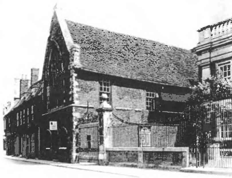
Fig 1 Boston Guildhall was built of brick with stone dressings in 1390 and just after and retains much of its original roof timbers under the reused medieval tiles on the south side.
