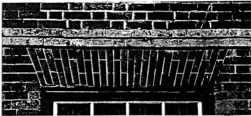
Fig. 2 Skewback with angle of 70°, Harwich, Essex
