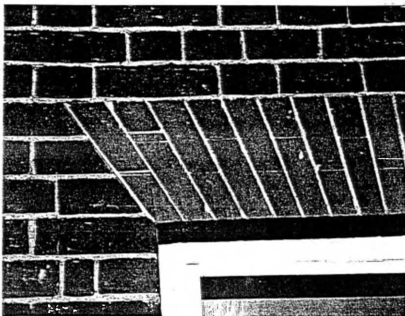
Fig. 1 Skewback, angle of 54°, Aldeburgh, Suffolk
