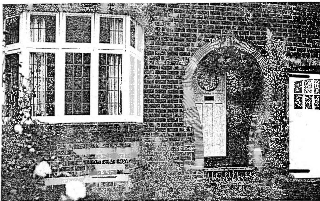
Fig. 3 Stretcher bond used on a bay-fronted house. The majority of semi-detached houses were built using stretcher bond. The porch is picked out by the use of tiles, which echo their use over the garage door. Individual details like this marked this house as different to its neighbours.
