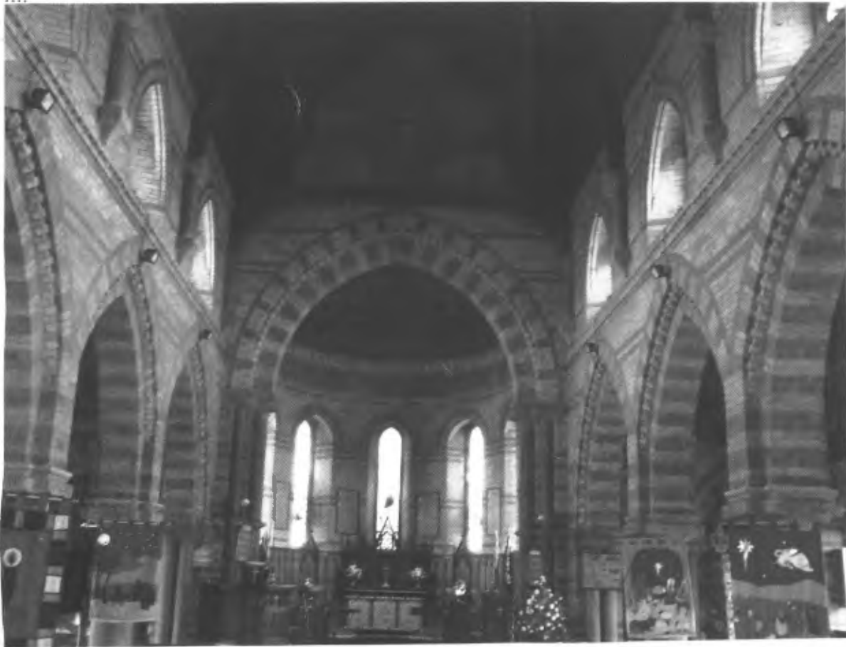
Fig.2 The chancel arch of Christ Church, Silloth, Cumbria, with the nave in the foreground and the apsidal chancel beyond was constructed in polychrome brickwork using red and yellow bricks.
