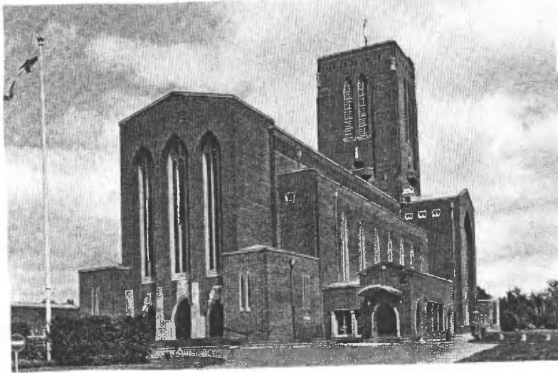
Fig.2 Guildford Cathedral, by Sir Edward Maufe, was built in two campaigns interrupted by the Second World War; it was consecrated in 1961 but work was not completed until 1966. The red brick is laid in Monk Bond.
