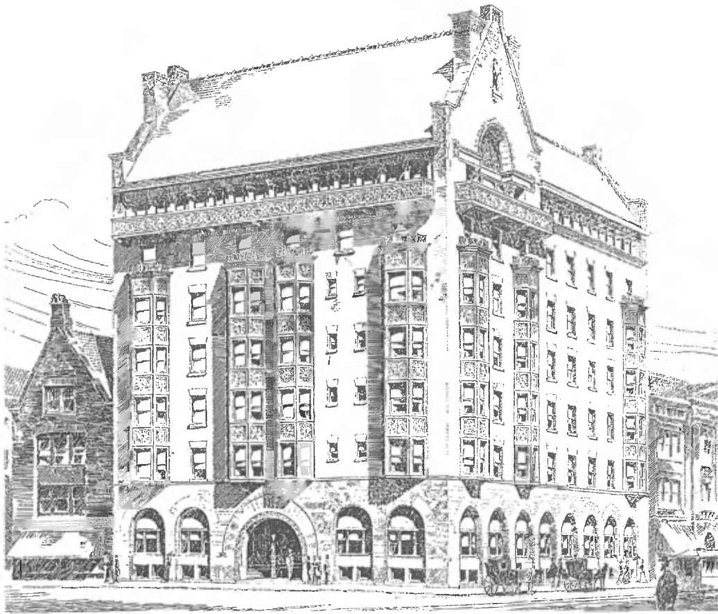
Fig.3 St Nicholas Hotel, St Louis, Missouri, USA (Adler & Sullivan, 1892-93, demolished). The terracotta on the ground and first floors, the bay windows and the seventh-floor balconies was supplied by the Winkle Terra Cotta Company. Building remodelled after a fire in 1903 and demolished in 1973. One set of the four panels making up the terracotta ornament on the bay windows is in the Sullivan Collection of the Southern Illinois University at Edwardsville, Illinois.
