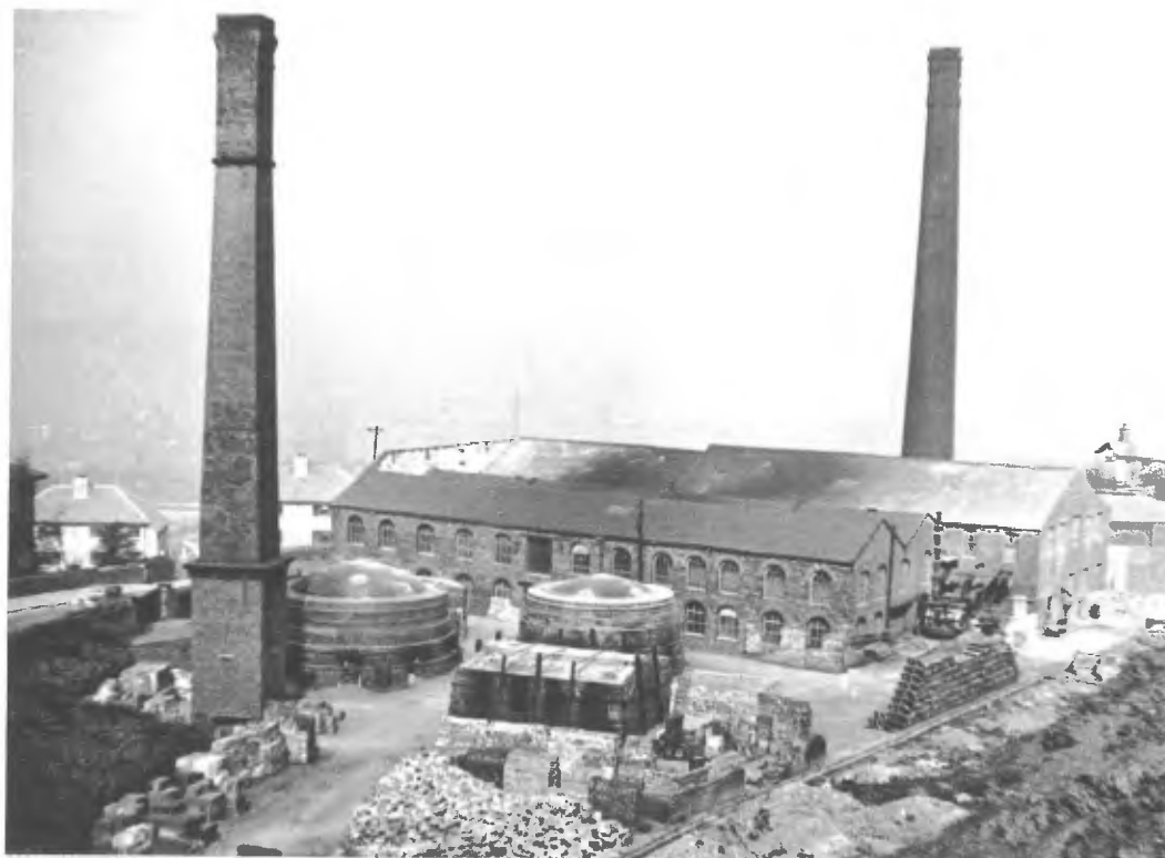
Fig.3 A local brickworks in operation at Wrose Hill, Shipley, in the 1930s. A Scotch kiln and two Beehive kilns are visible in the foreground. Mapping evidence indicates that the chimney in the background forms part of a Hoffman kiln.
