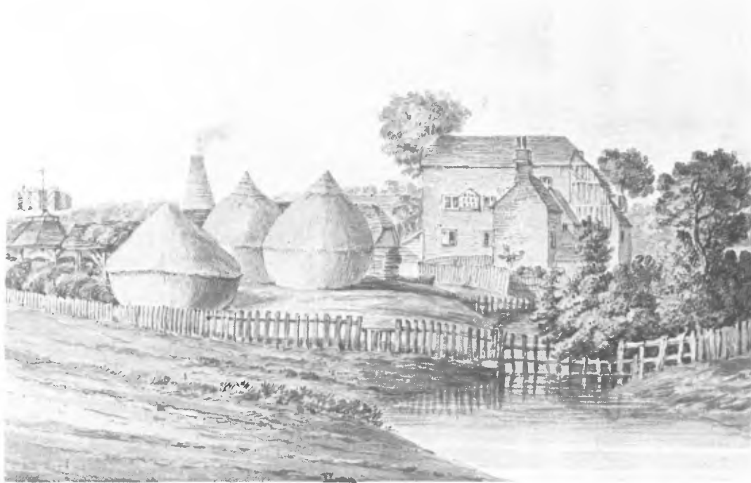
Fig. 1 The brick kiln at Crawley Mill, Husborne Crawley, Bedfordshire, where the tilemaking machines developed by Robert Beart, the Marquess of Tweeddale, and William Irving were all tried, those by Beart and Tweeddale being the most successful. The kiln is left of centre behind the haystacks, with the drying sheds to the left of the haystacks and the wind-driven clay mill on the extreme left. Motive power for clay mill could also be provided by using one or two horses. This was the estate brickyard and one of the estate corn mills for the Duke of Bedford's estate in central Bedfordshire based on the parishes adjacent to his house and park at Woburn Abbey.
