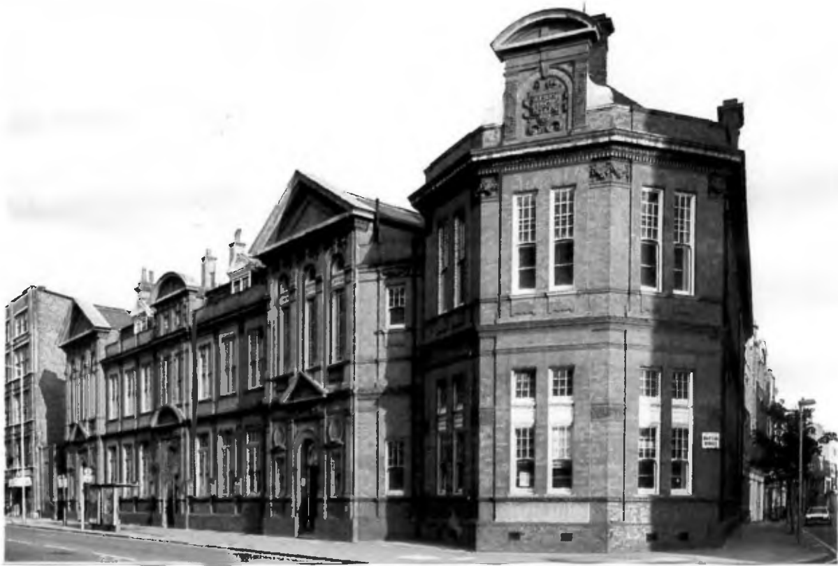
Fig. 1 The Offices of the Board of Guardians of Holborn Poor Law Union, Clerkenwell Road, London EC1, built in 1886 to the designs of H. Saxon Snell & Son, using blue brick in the lowest courses and a fine orange-red brick from the window sills of the ground floor upwards. The arms of the organisation appear under the segmental pediment above the wide canted bay at the right.
