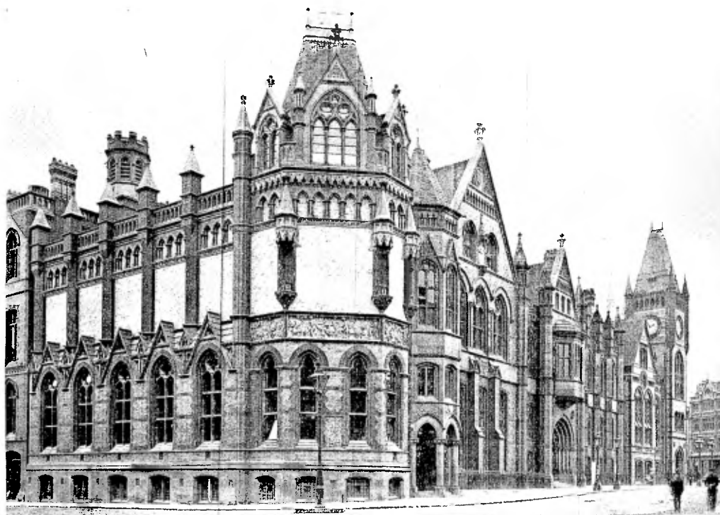
Fig. 2 Reading Town Hall, a photograph taken soon after the complex was completed in 1897. This photograph brings out the very light colour of the bricks used on the first floor of the Art Gallery, erected 1896-7, centre left, in contrast to the much darker brick used on the 1879-82 portions, centre right and extreme left. As can be seen, economy was exercised by not filling the niches at the corners of the canted bay and leaving uncarved the band of sandstone blocks on the Blagrove Street front.
