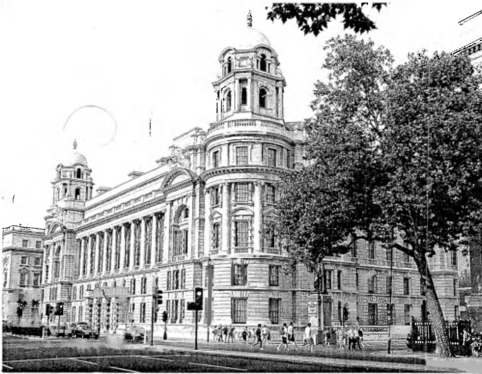
Fig. 4 The New War office from the south, showing part of the frontage to Horse Guards Avenue (partly behind the tree) and the drum tower at the corner. Contemporaries criticised the use of Doric columns on the drum towers and cupolas above the Ionic columns of the main façades.
