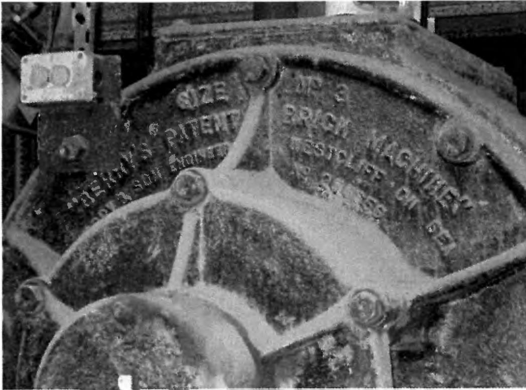
Fig.2 Berry's Patent Brick Machine
