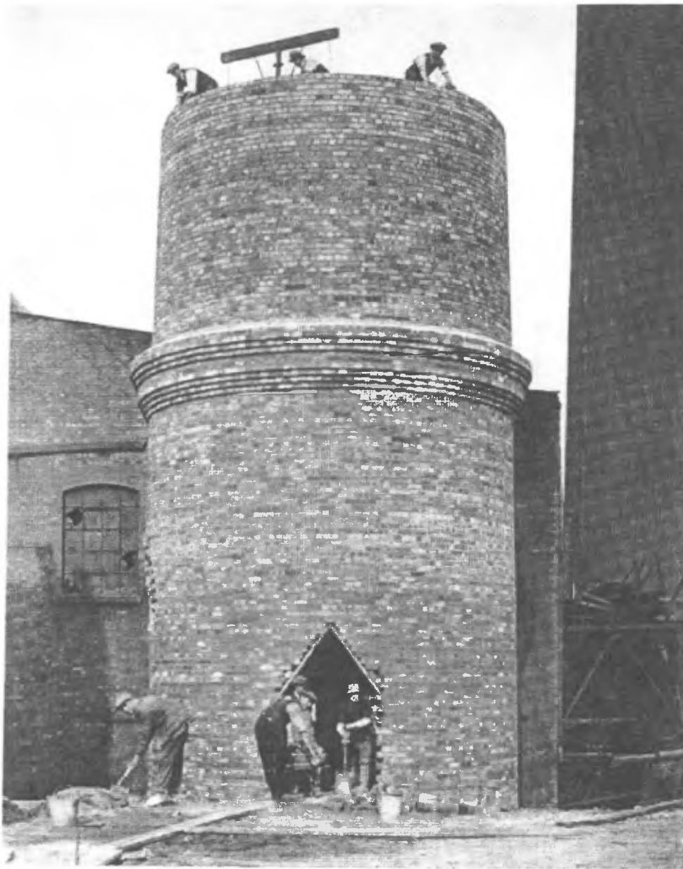
Fig. 2 A chimney shaft in the course of construction.
