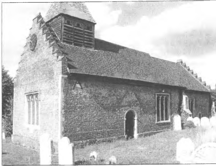
Fig. 2. Woodham Walter Church. This church has conventionally been dated to 1562-1564 based on documentary evidence and a date plate within the church. However, dendrochronology undertaken on the timbers in the belfry produced a late-fourteenth-century date, suggesting a re-cycling of materials had taken place and highlighting a potential limitation to dendrochronology.
