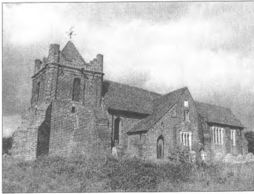
Fig. 1 East Horndon Church. Documentary sources indicate that the main body of the church was built by c.1476 and that the south chapel was built c.1510. However, there is no record of when the south porch was added. A multi-phased brick structure such as this presents an opportunity to evaluate the ability of luminescence to date different brick parts, a task that can be challenging to current brick typologies.
