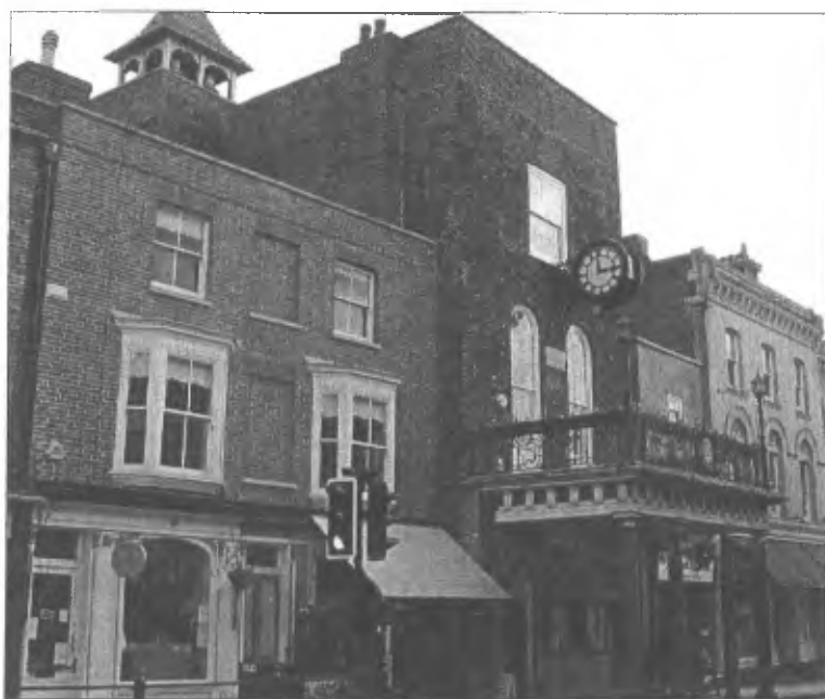
Fig. 4. The Moot Hall, Maldon. Built in the early fifteenth century, the structure incorporates a number of rare and unusually early brick features, including a brick newel staircase and trefoil corbelling made from carved bricks.
