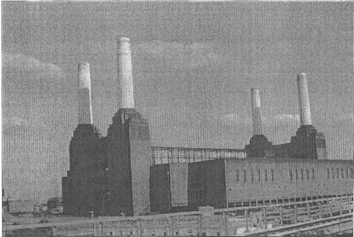
Fig. 1. Battersea Power Station from the west, with the River Thames on the left. The photograph shows the exterior of the western turbine hall and the central boiler house with the four white chimneys. The decorative use of brick on the upper parts of the unpainted sections of the chimney stacks is clearly visible as is the unroofed nature of the central portion of the structure.
