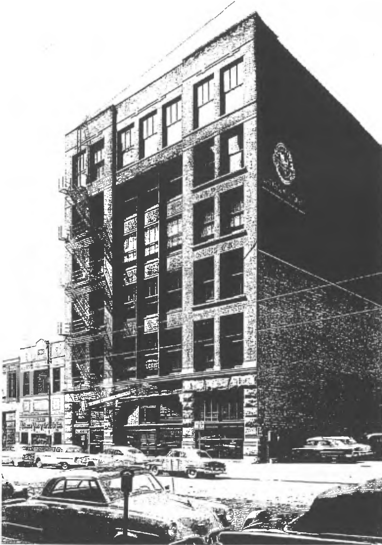
Fig. 3 The Wirt Dexter Building, 630 South Wasbush Avenue, Chicago, of 1887, which in 2006 was about to be refurbished. This is one of only three early Sullivan office buildings where the brick is load-bearing to survive. The top floor is a later addition which accounts for the survival of the brick cornice above the fifth floor. The first floor (American; ground floor in English) is clad with granite.
