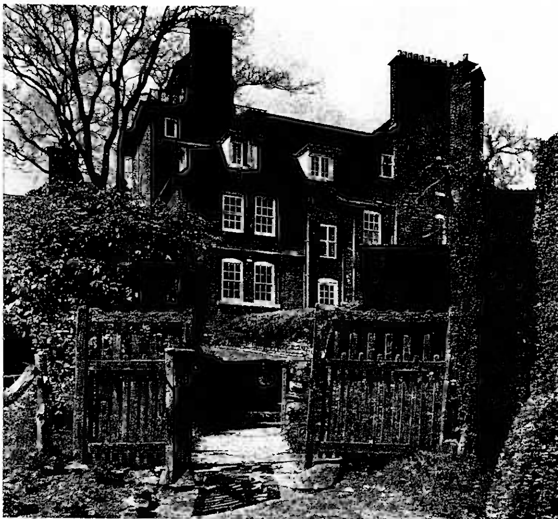
Fig. 1 A portion of the east front of 'Standen'. This is the maximum use of brick on the exterior but the two left-hand windows of the first floor are set within a tile-hung portion of the wall. The big chimney stacks are brick but the water tower is rendered.
