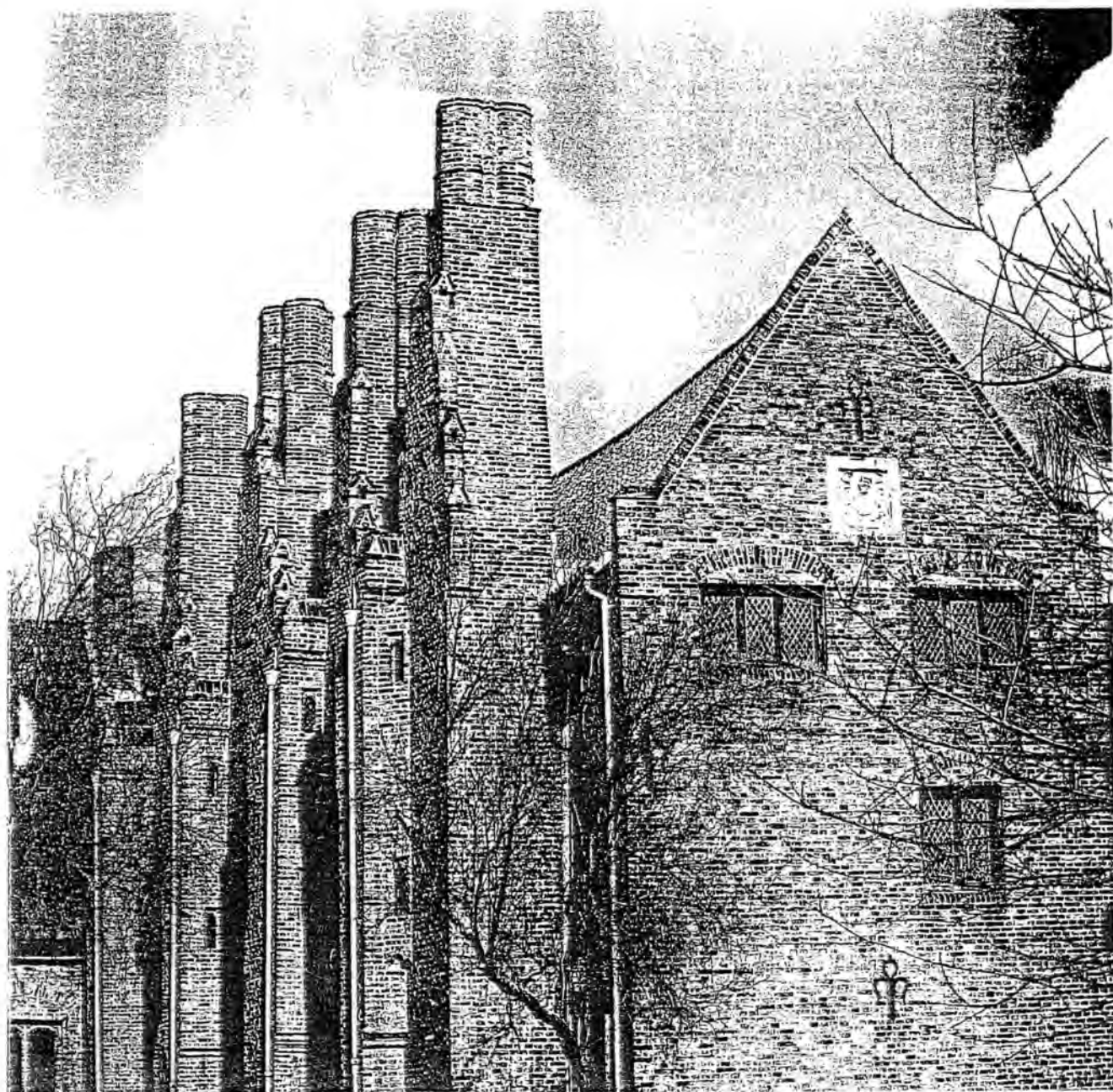
Fig. 2 Gainsborough Old Hall: the west wing showing the garderobe towers with attached chimneys of the 1470s and a south gable of c.1600.
