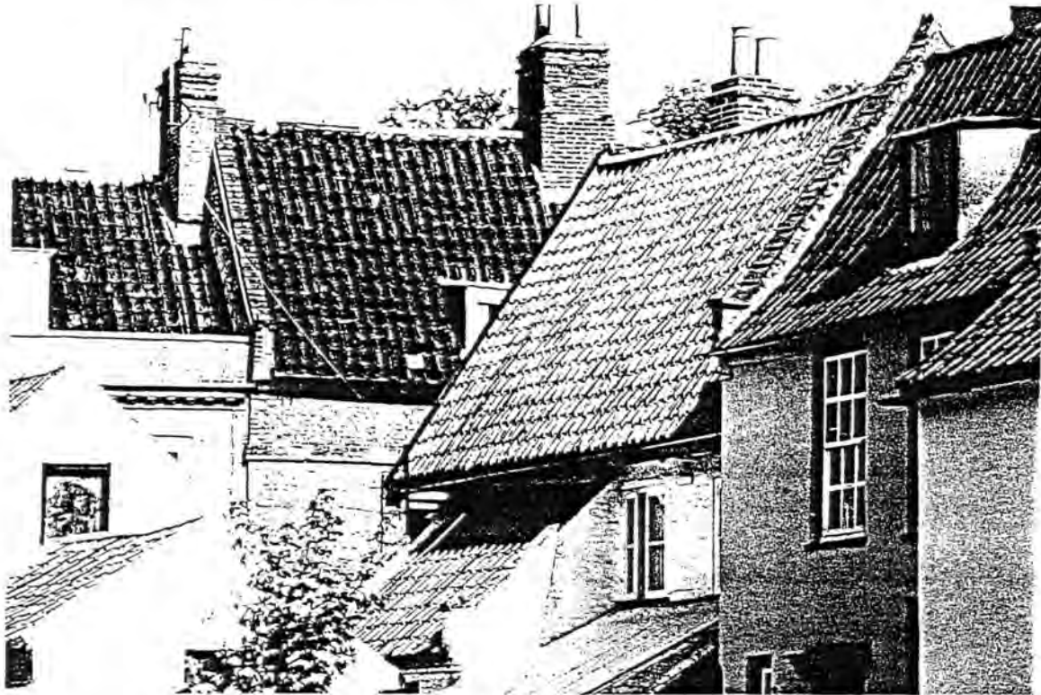
Fig. 1 Rebated Coping Tiles on buildings at Little Walsingham, Norfolk.
