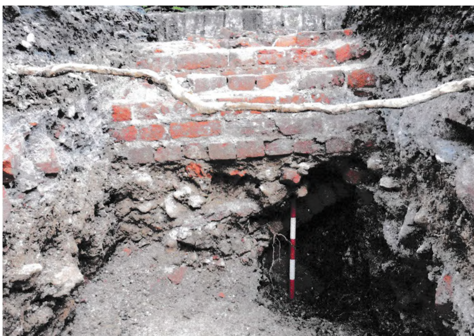
Fig. 1 View of the reverse arches at Kearnsey Park, Dover, Kent, under excavation.
