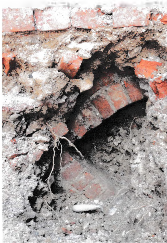
Fig. 2 The reverse arches at Kearnsey Park, Dover, Kent, visible in the excavation trench.
