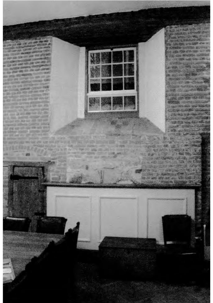
Fig. 10 (right) Window in north wall note the infilling below and the cut bricks to the left reveal.
