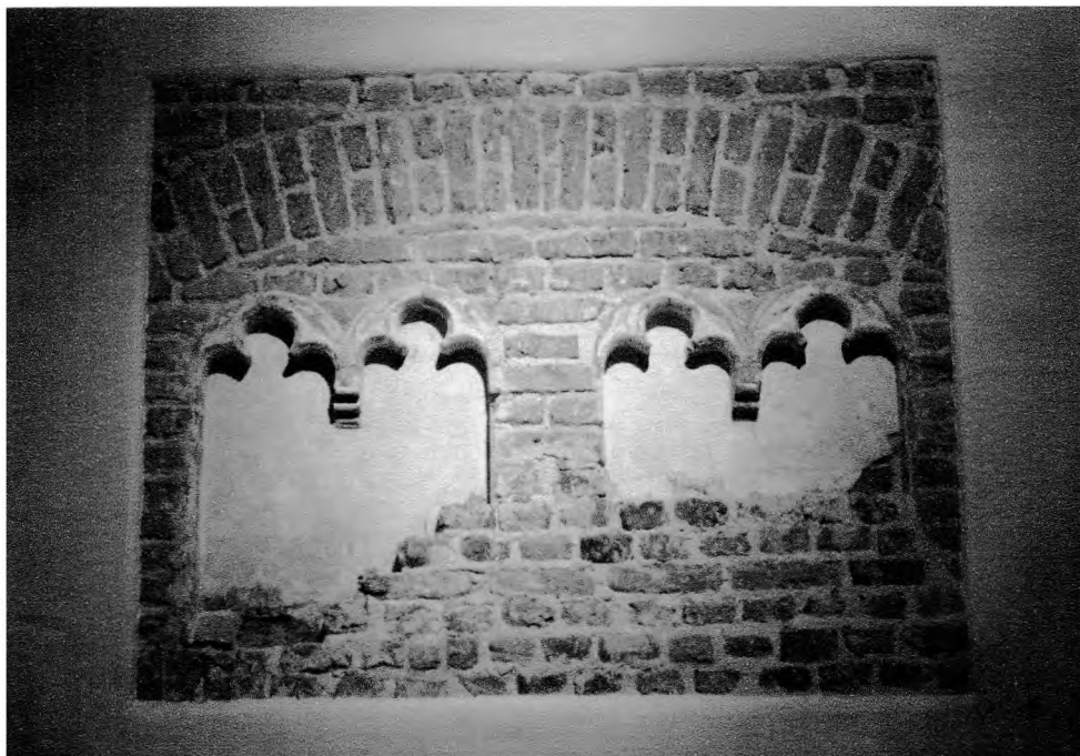
Fig.16 The trefoil headed arches of the first floor chamber fireplace.
