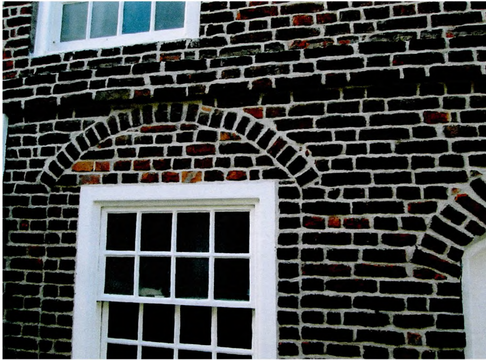
Fig. 3 View showing infill around the ground floor window of Fisherman's Cottage, Deal,
